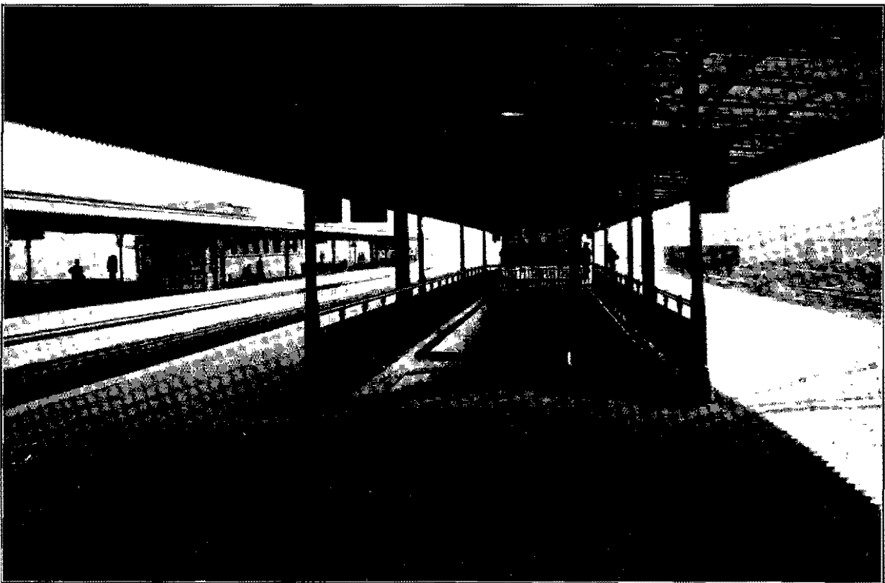
ONE OF THE TWO NEW "ISLAND" PASSENGER PLATFORMS AT SPENCER-STREET FOR SUBURBAN TRAFFIC. Length, 520 feet. Served by 30 feet wide subway, which, with buildings, is faced with tiles to facilitate cleaning and to improve appearance (See page 20.)
