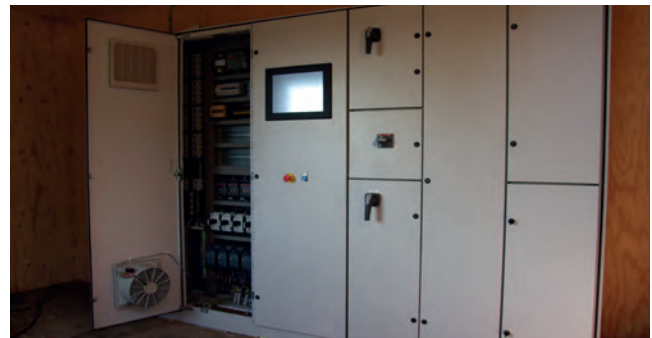
Silo installation with a shed for control panel, distribution board and enough space for a table for crop analysis equipment etc. You can easily inspect the space and intake pit.
