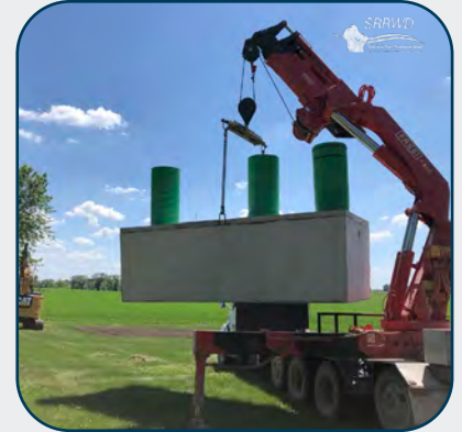
Septic tank install
