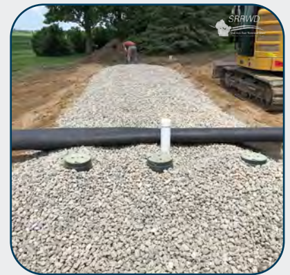
Mound septic system construction
