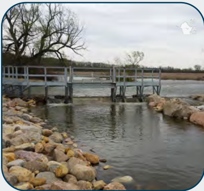
Pickerel Lake Dam
