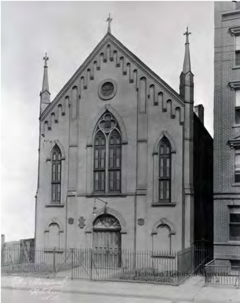
Figure 6. Photograph of the ca. 1879 German Methodist Church/St. Matthew's Baptist Church at 131-133 Garden Street (Property ID 618181867; locally designated) in 1933. Note the similarities between 637 Garden Street (Source: Hoboken Historical Museum).
