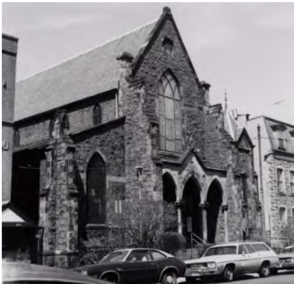
Figure 12. View of the resource northwest from Hudson Street in 1976, just prior to its residential conversion (Source: Hoboken Historical Museum).
