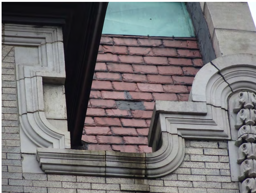
Photograph 7. Detail view of the roof of the building; view east.
