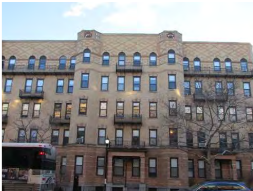
Photograph 4. Looking at the west elevation of the south half of the complex, view east.
