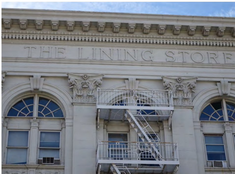
Photograph 9. Detail view of the ca. 1915 terra cotta "THE LINING STORE" lettering below the cornice on the primary elevation of the building.
