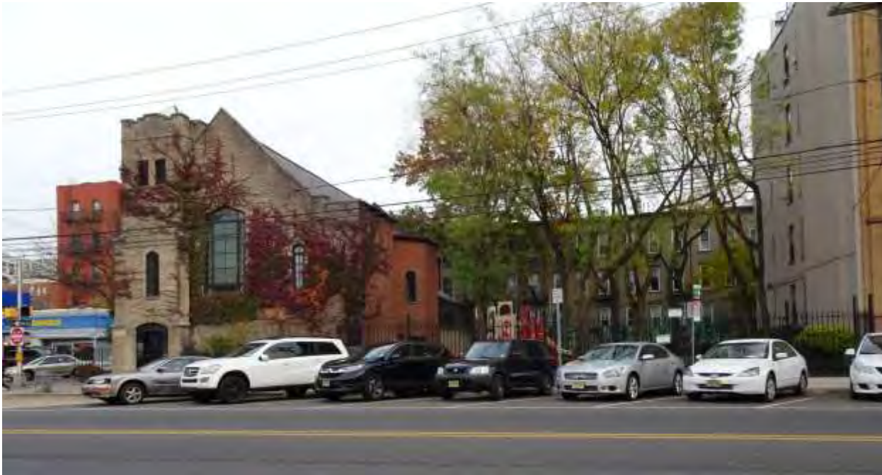
Photograph 11. The former Norwegian Church situated along the Willow Avenue streetscape, view northeast.
