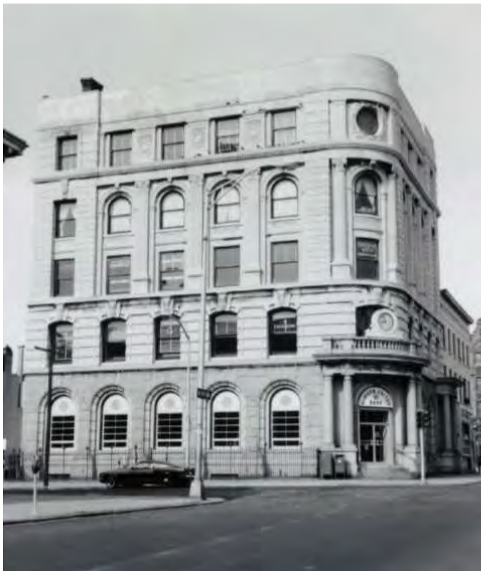
Figure 10. View of the Hudson Trust Building in the 1970s, when the company was renamed Hudson United Bank. Despite the retained integrity, the roofline at this point had lost its characteristic balustrade (Source: Hoboken Historical Museum).
