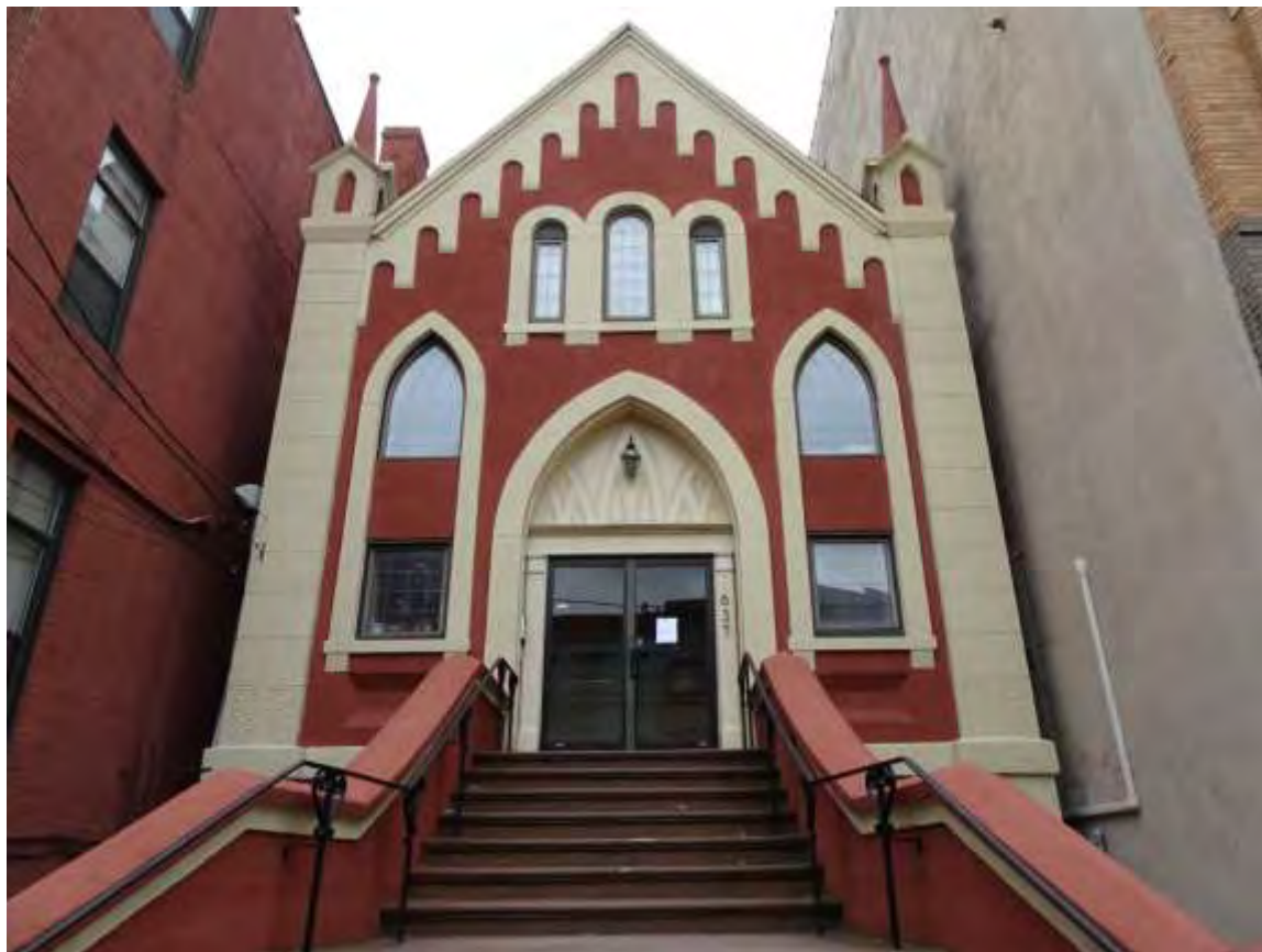
Photograph 1. Primary elevation of the former Temple Adath Emuno, view east.
