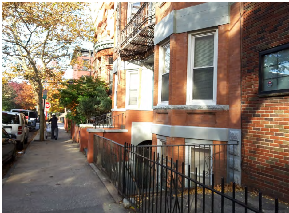
Photograph 6. Street-level view of the garden level access of the Marguerite apartment building looking west.
