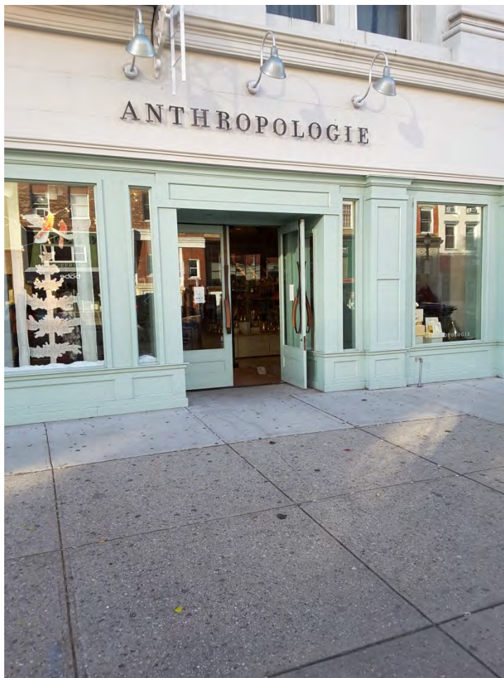
Photograph 3. View of the modern storefront on the Washington Street elevation of the building at 412 Washington Street.
