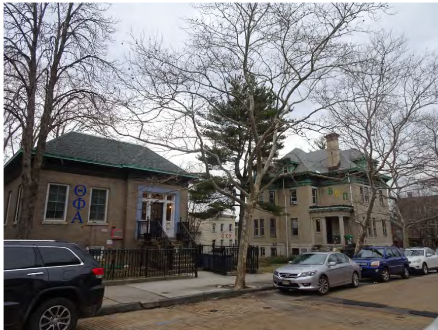
Photograph 4. View northwest along the 800 block of Castle Point Terrace showing, from left to right, 808 Castle Point Terrace and 812 Castle Point Terrace.
