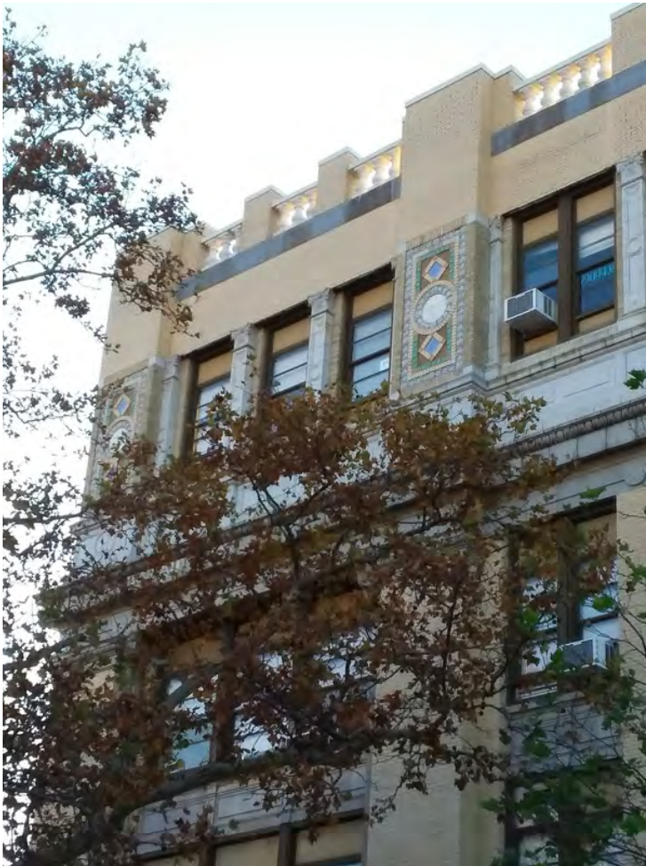
Photograph 7. Detail view of the fourth floor, view northwest.
