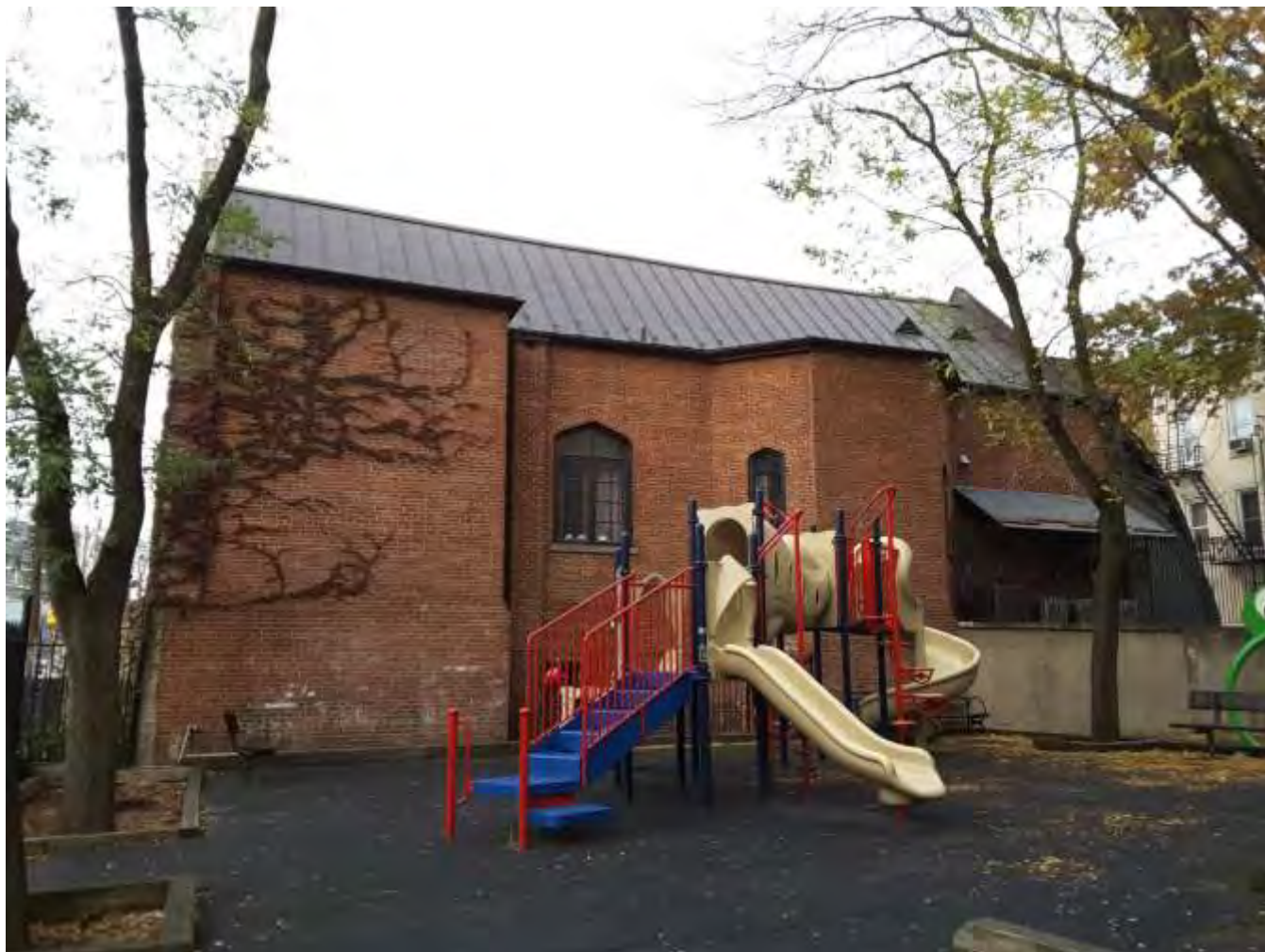
Photograph 5. View of the south elevation, looking north from Legion Park.
