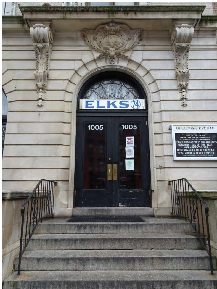
Photograph 2. Looking at the main entrance along Washington Street, view east.
