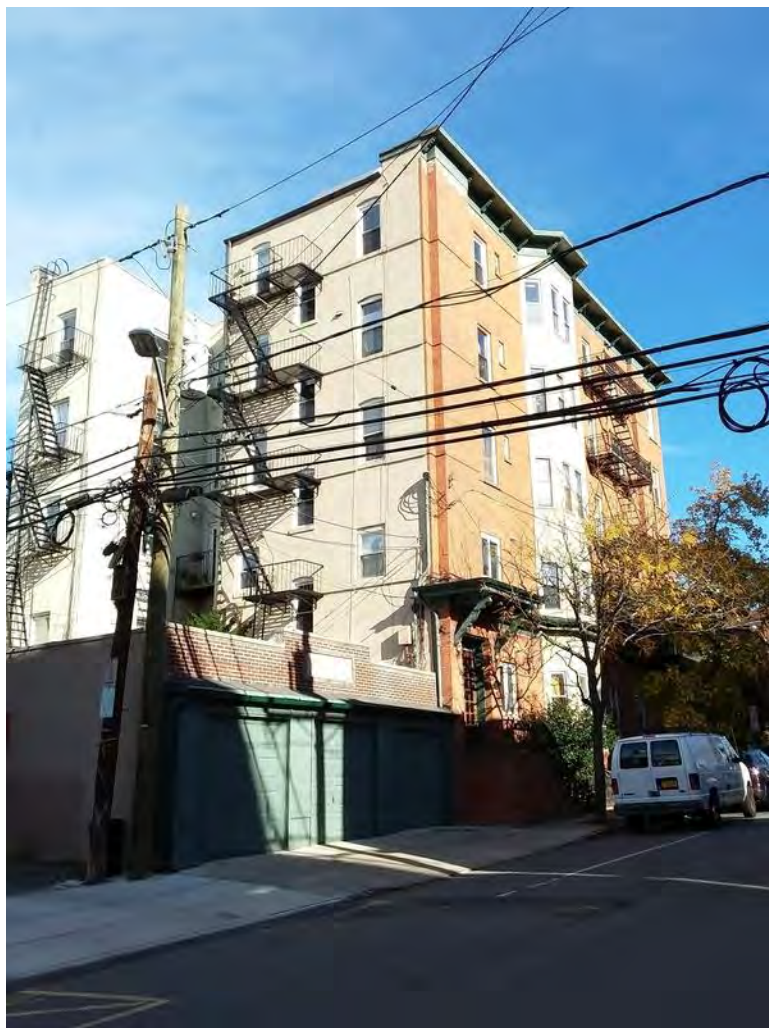
Photograph 3. 500 Hudson Street's south elevation and rear (west elevation), showing one-story garage attachment, view northeast from Fifth Street.
