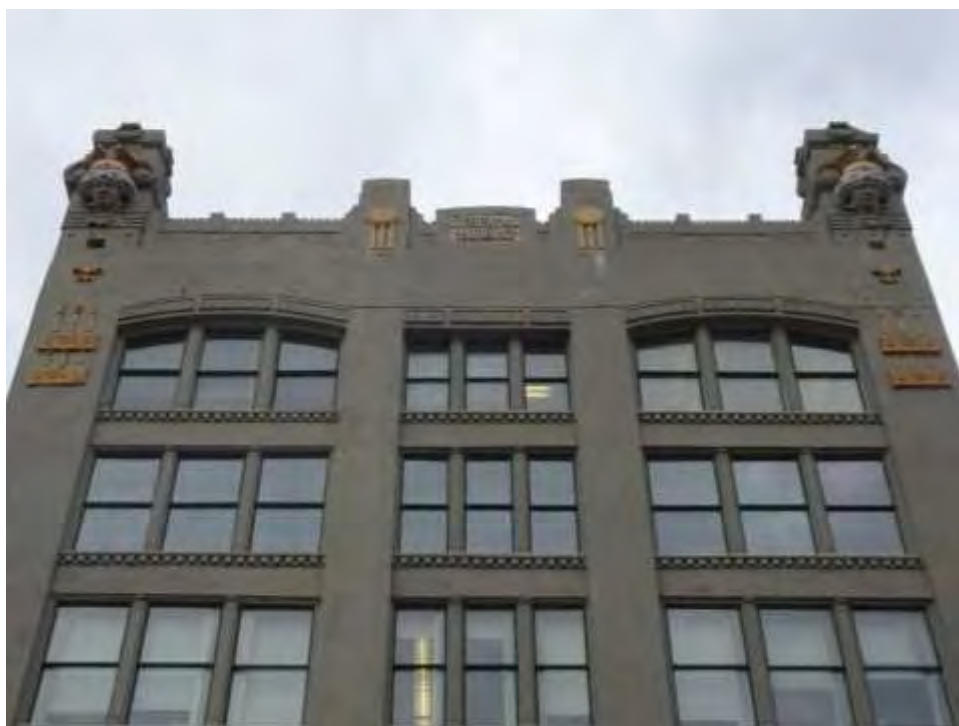
Photograph 4. Detail view of the cornice, view west.
