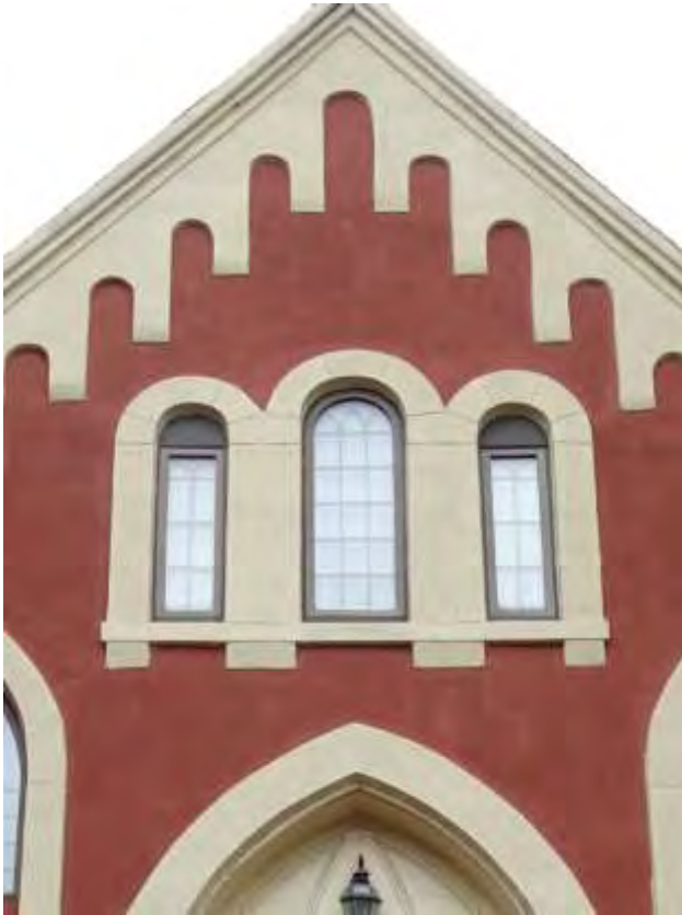
Photographs 5, 6. Replacement sash set into original openings, replacing significant stained glass elements.
