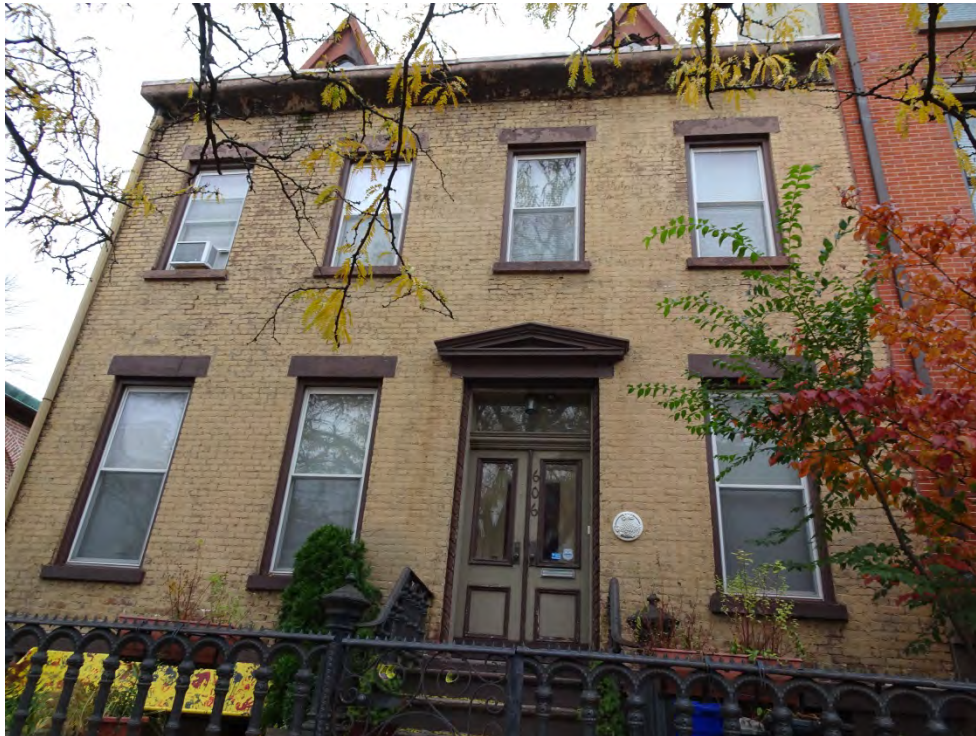
Photograph 5. Looking at the façade of the rectory building, sited north of the church building, view west.
