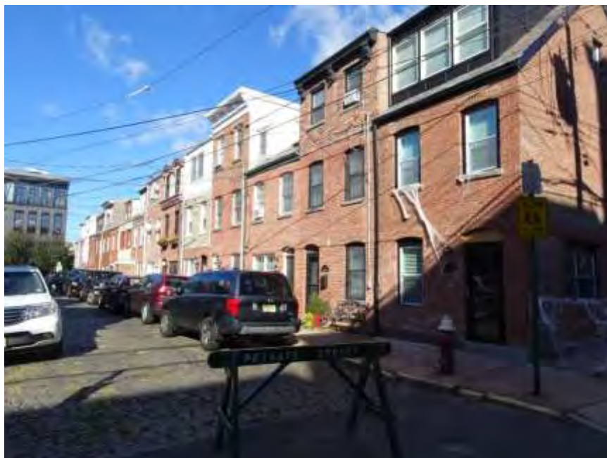
Photograph 3. View north of the north side of Willow Court South, from Willow Avenue.
