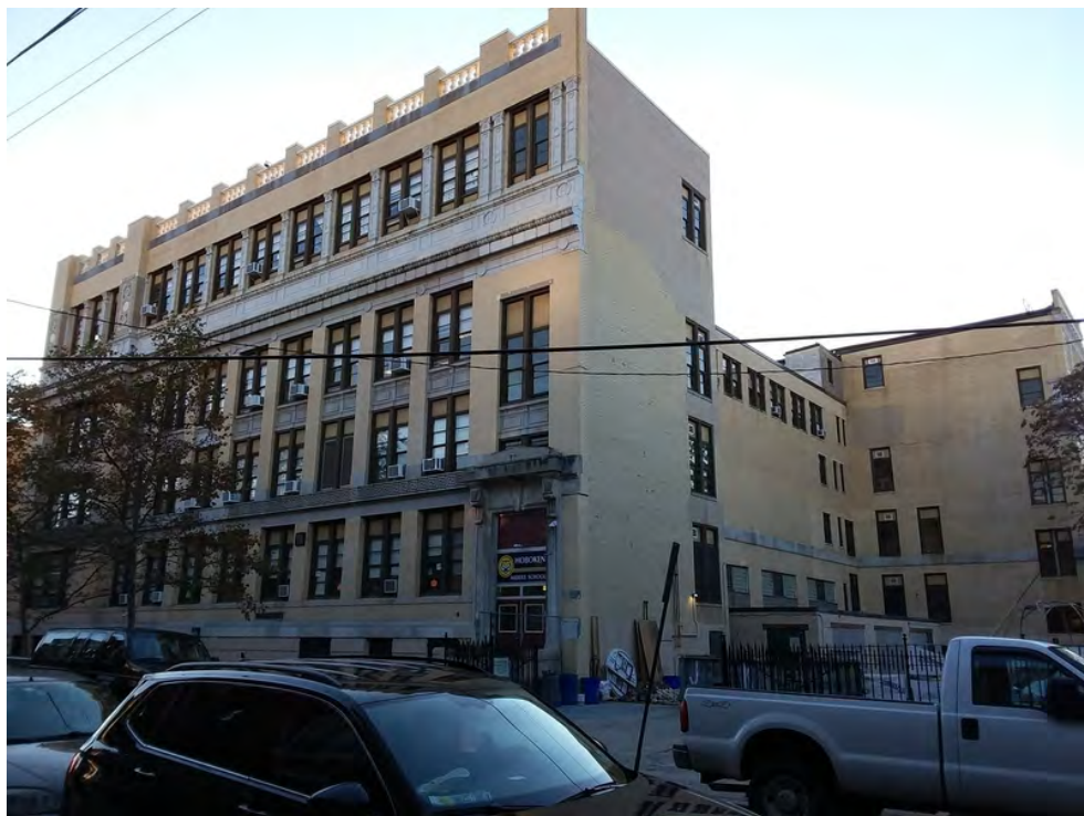
Photograph 5. Looking at the east and north elevations of the building, view southwest.
