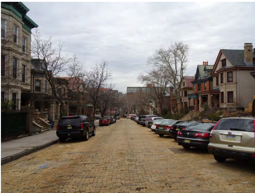
Photograph 12. View north along the 900 block of Castle Point Terrace from Ninth Street.
