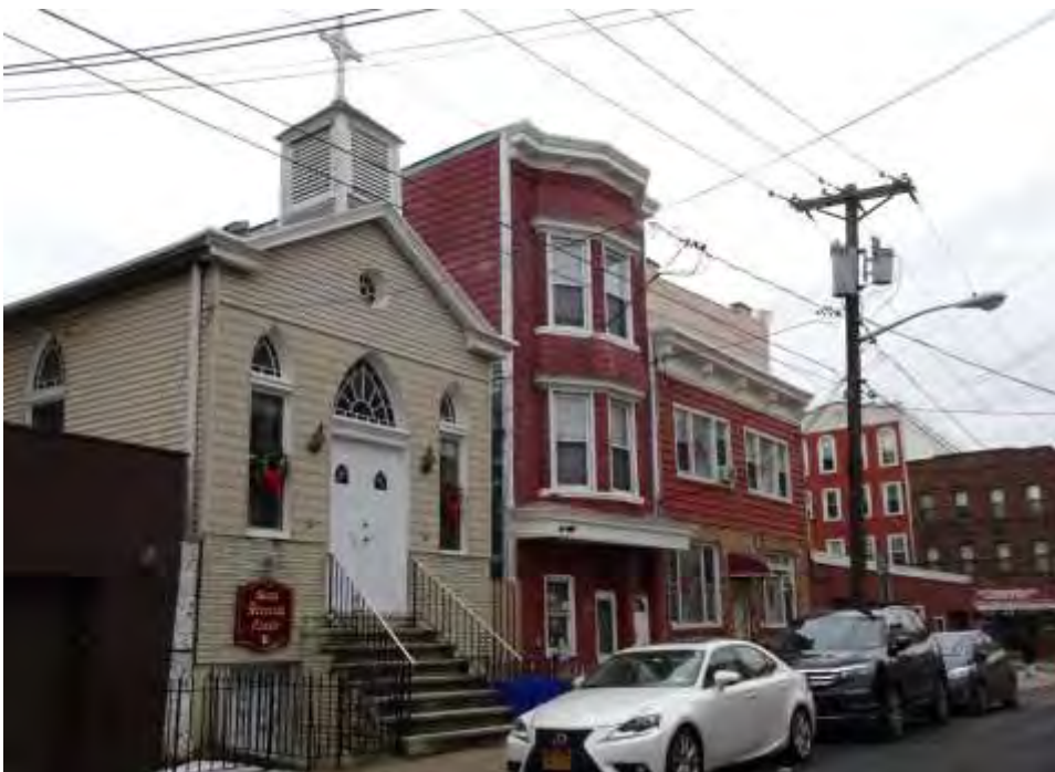
Photograph 3. Southwest view of the chapel situated on Fifth Street.
