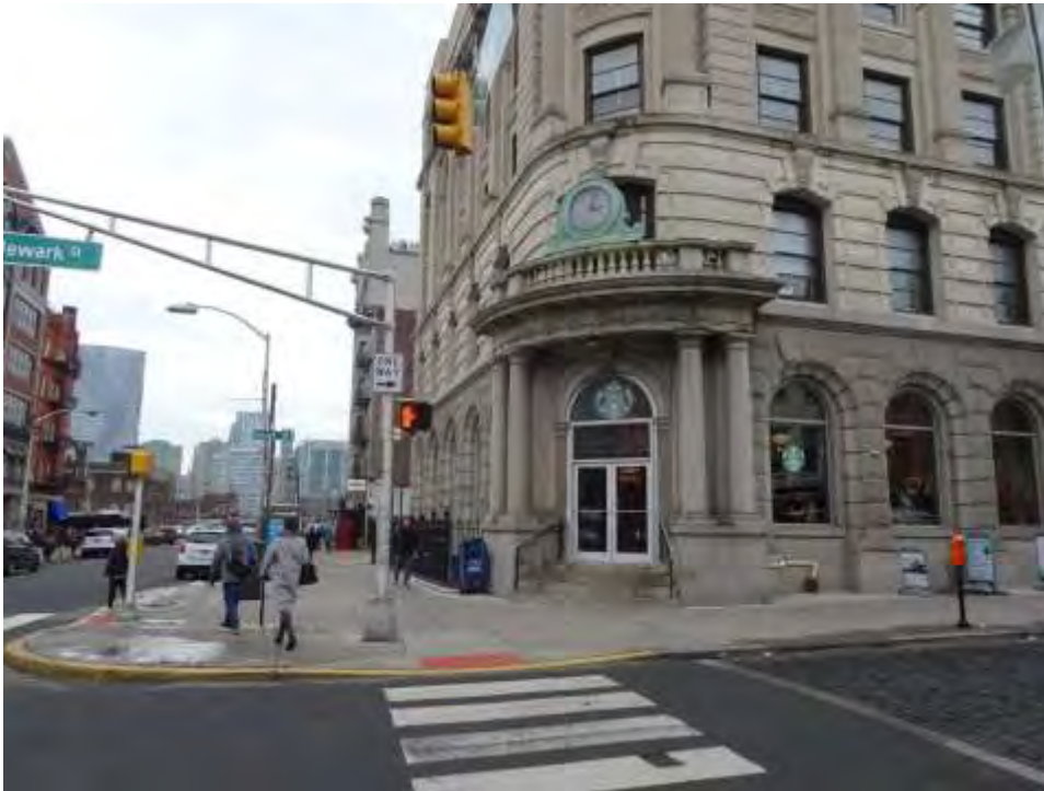
Photograph 8. Hudson Street streetscape, view south from Newark Street.
