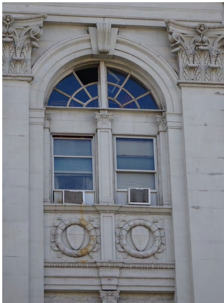
Photograph 5. Detail view of historic terra cotta detailing on the primary elevation of the building as well as ca. 1985 fanlight transom.
