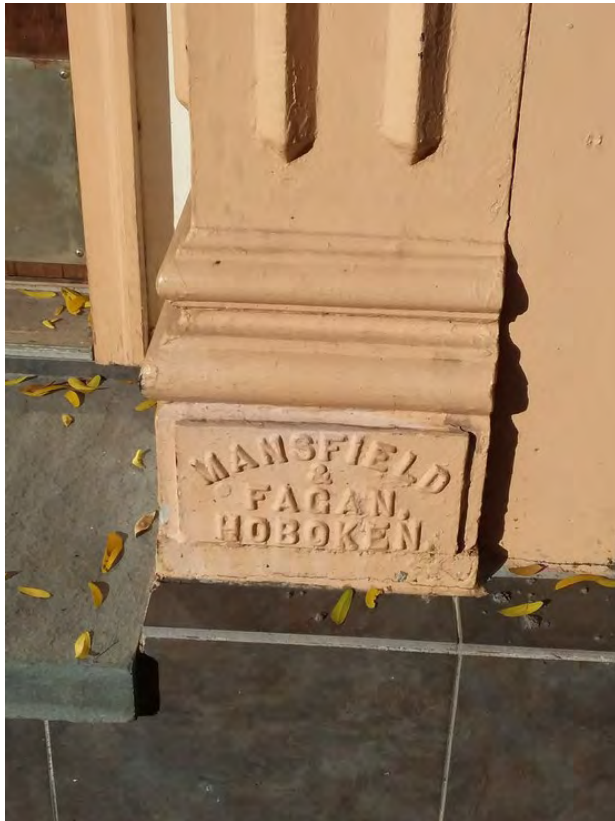
Photograph 6. (left) Visible manufacturing mark of Mansfield & Fagan Architectural Iron Works at 700 Washington Street, whose marks remain visible at the base of many cast iron storefronts throughout the Washington Street Corridor.
