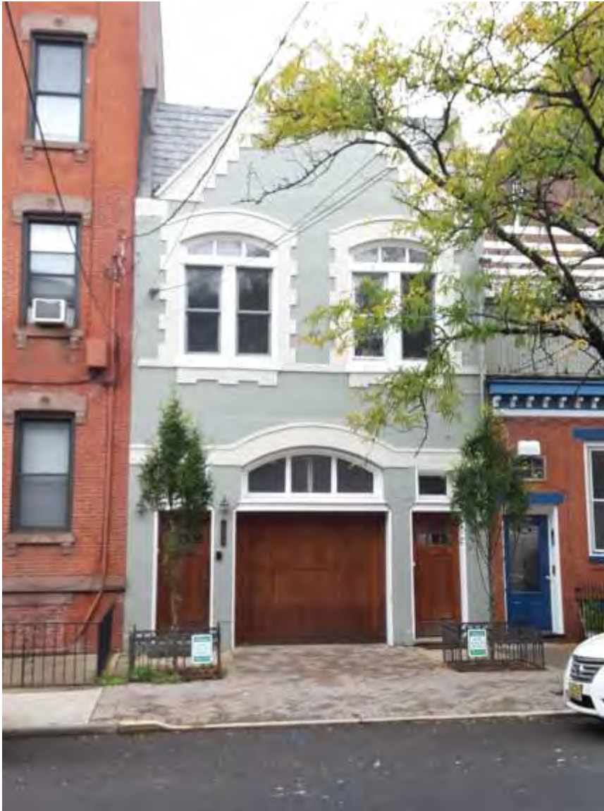
Photograph 1. 1028 Willow Avenue's primary elevation, view west from Willow Avenue.
