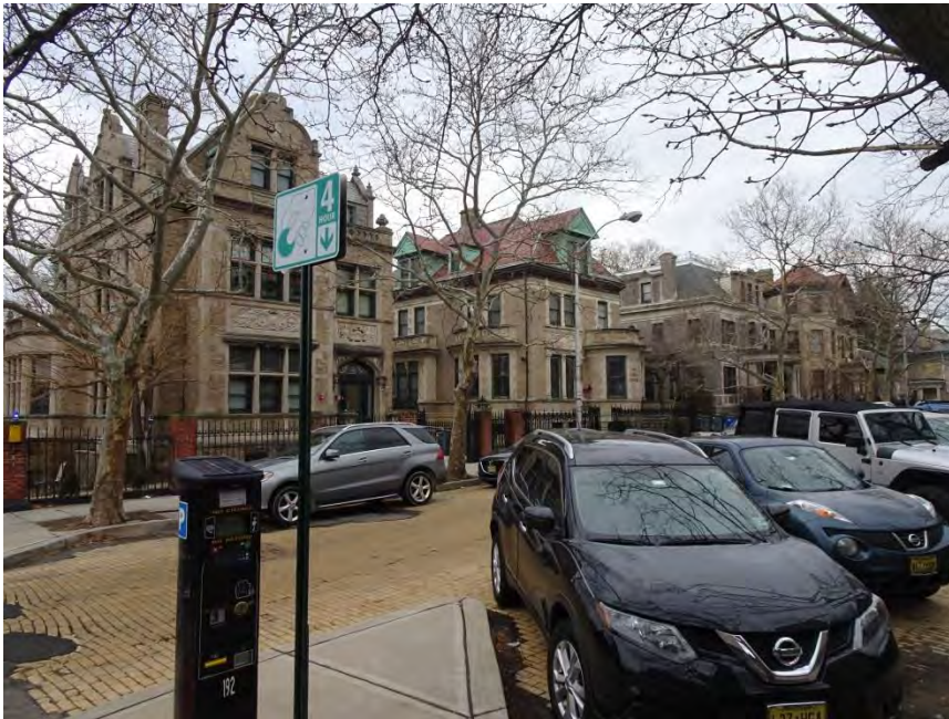
Photograph 11. View northwest along the 800 block of Castle Point Terrace showing, from left to right, 800, 802, 804, and 806 Castle Point Terrace.
