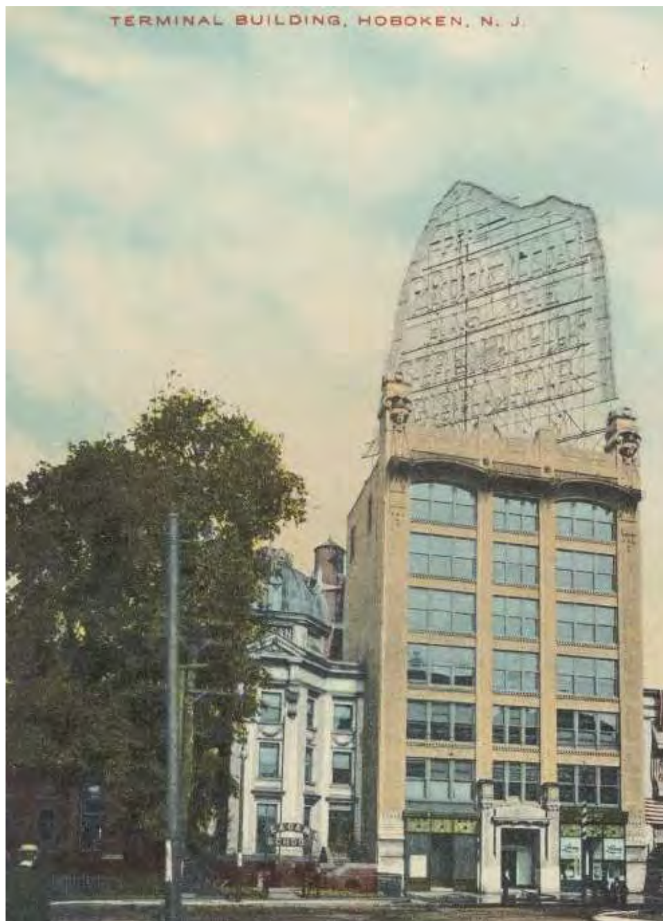
Figure 4. Postcard rendering of the Terminal Building, recording the Prudential Insurance Rock of Gibraltar sign, ca. 1911-1915 (Source: Hoboken Historical Museum).
