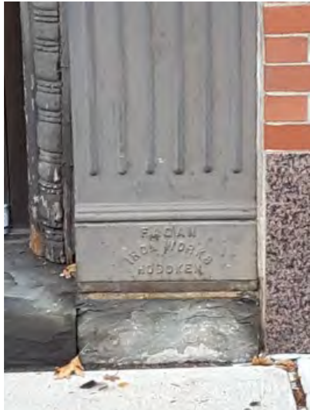
Photograph 6. (left) Visible manufacturing mark of Mansfield & Fagan Architectural Iron Works at 700 Washington Street, whose marks remain visible at the base of many cast iron storefronts throughout the Washington Street Corridor.
