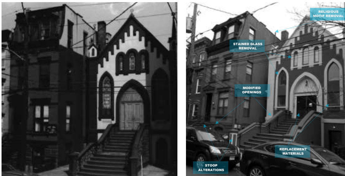
Figures 9, 10. Side-by-side comparison of the former Temple Adath Emuno and 639 Garden Street, illustrating four decades of change from 1978 (left) and 2019 (right) (Source: NJ HPO; AECOM).
