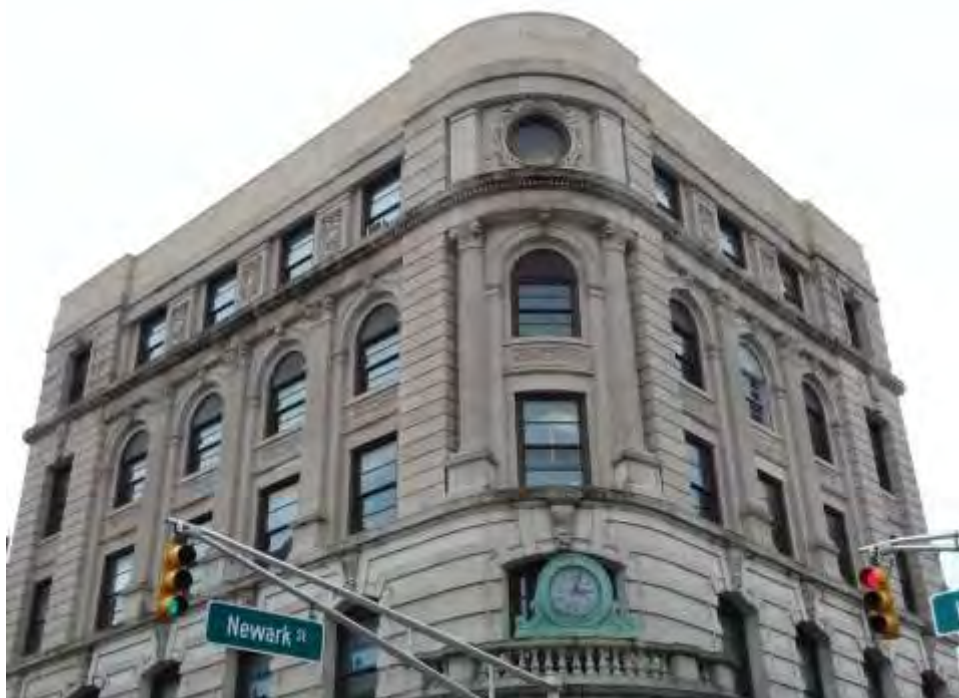
Photograph 7. View of the adapted balustrade, looking southwest.
