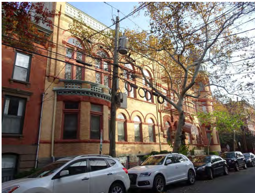
Photograph 2. Looking at the façade along Bloomfield Street, view southeast.
