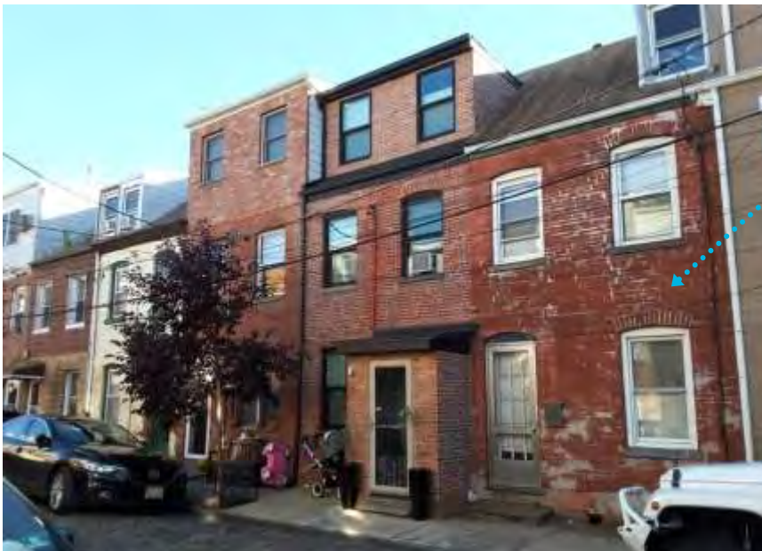
Photograph 2. View southeast of the south side of Willow Court South, from Clinton Street. Note 29 Willow Court, which stands as one of the best expressions of the original Willow Terrace rowhouses with its original window and door openings, roof, offset shared dormer, and bluestone threshold and sills.
