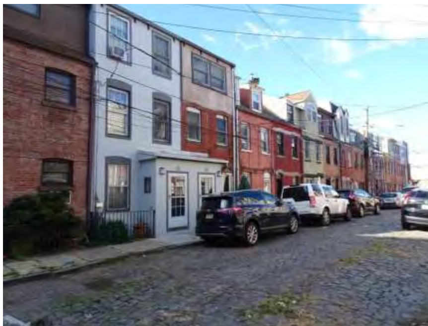
Photograph 4. View southwest of the south side of Willow Court North, from Willow Avenue.
