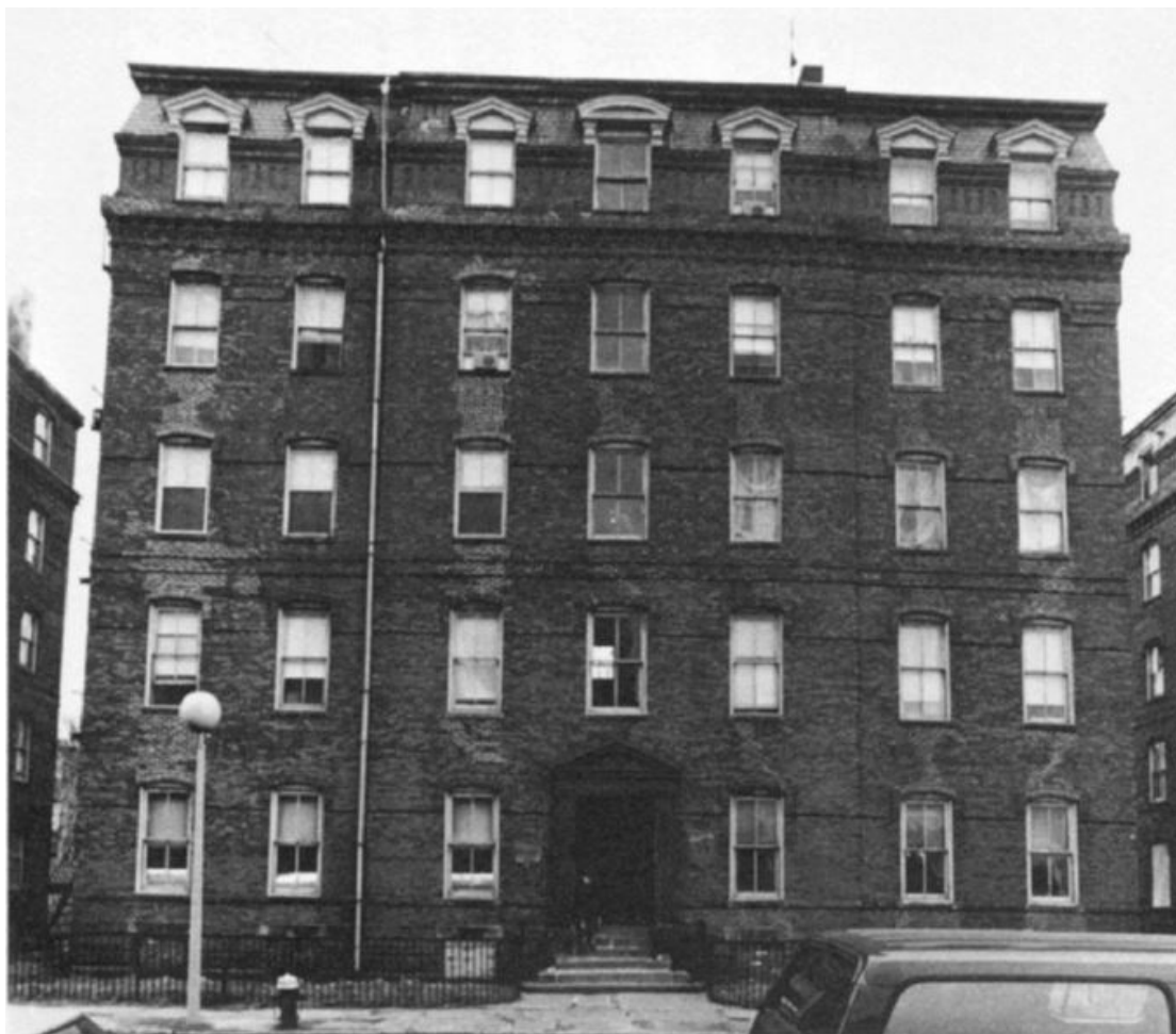
Figure 9. The Bigelow model tenement at 99 East Canton Street, Boston. The designed by Charles K. Kirby and erected in 1874-1875 by the trust established by Abbot Lawrence, it is a possible inspiration for the Odenheimer House (Source: Photograph by Barry Cohen, featured in Zaitzevsky, 1983:164).
