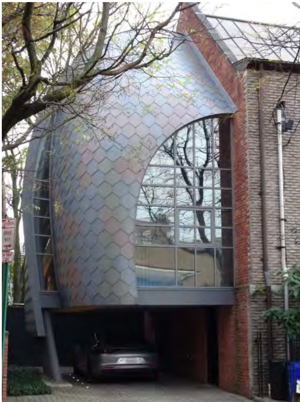
Photograph 7. Elevation of the modern apse annex affixed to the rear of the historic church, view south.
