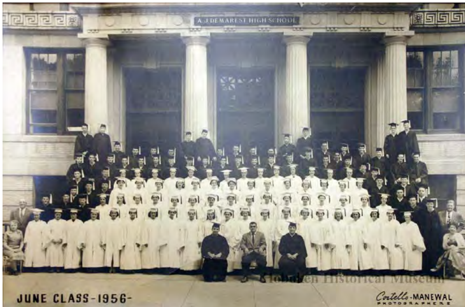
Figure 9. Image of the graduating class of 1956 in front of the main entrance of the school shows the original columns and entablature that have been removed. Photograph also shows transom panels that are still present above these doorways (Source: Hoboken Historical Museum).
