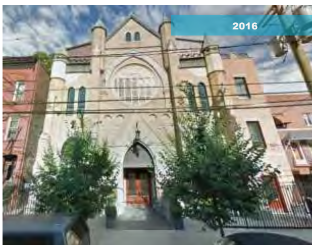
Figures 12, 13, 14. Adaptive reuse of the structure, as seen through Google Streetview from 2007-2016 (Source: Google).
