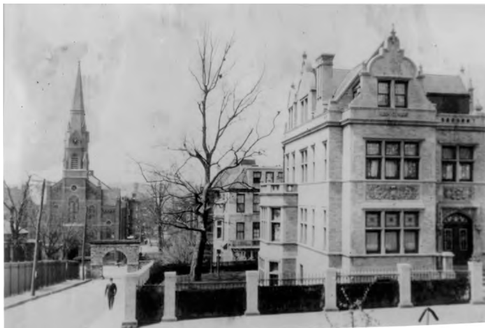
Figure 15. Early 20 th century photograph depicting the northwest corner of Castle Point Terrace and Eighth Street. 800 Castle Point Terrace is to the right of the photograph (Source: Rutgers University).
