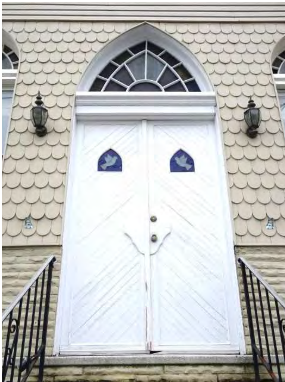
Photograph 4. View of the main entrance to the chapel, facing south.
