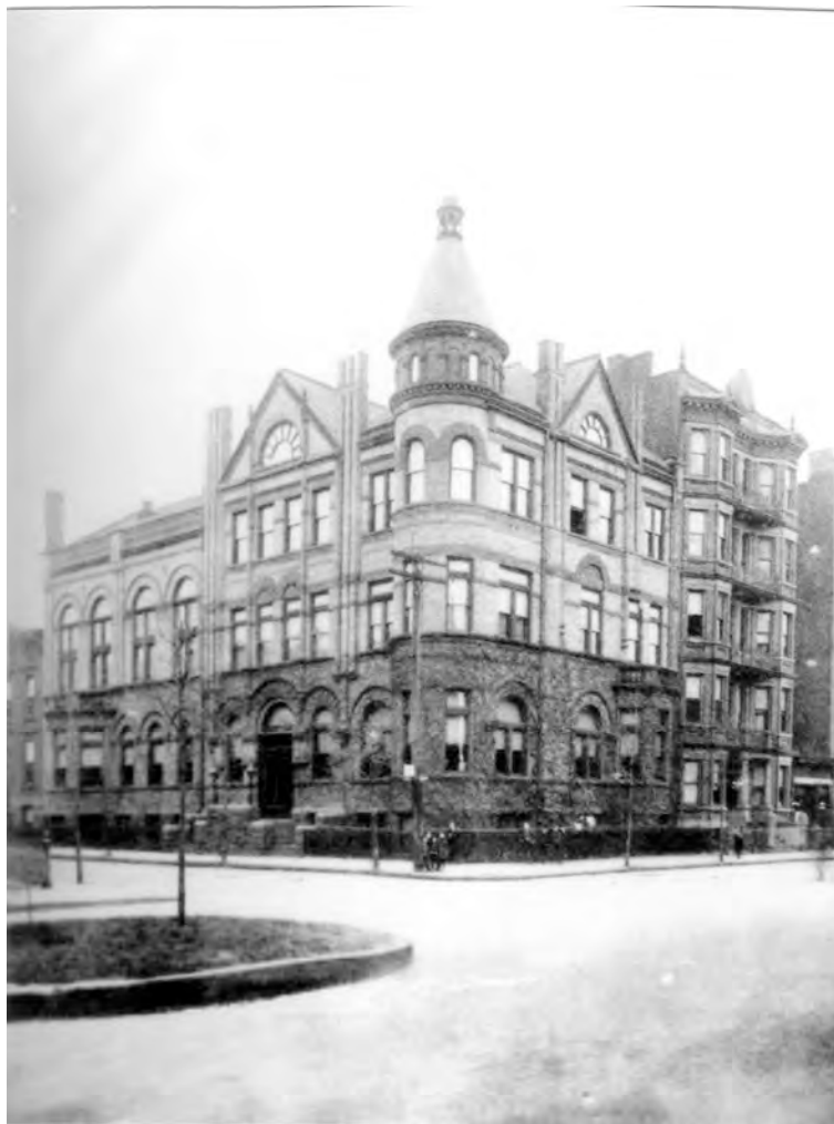
Figure 7. Documentation of the Columbia Club at 1101 Bloomfield Street ca. 1910 (Source: Rutgers Library).
