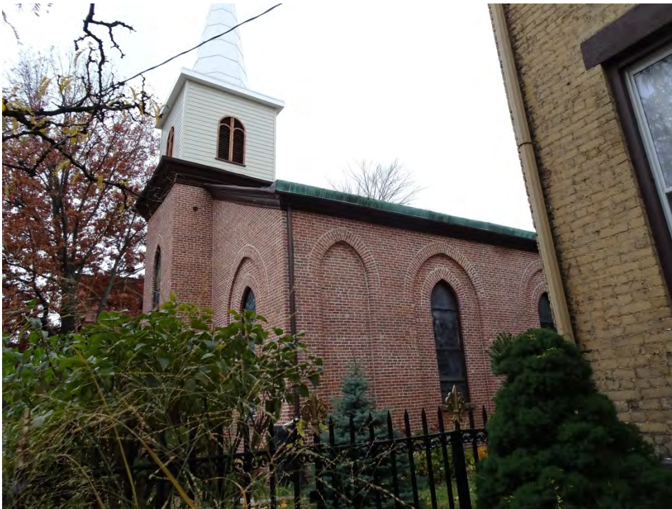
Photograph 3. Looking at the façade and north elevation of the Community Church of God, view southwest.
