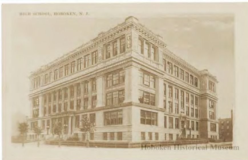
Figure 6. Postcard image of the school building after the fourth floor addition was constructed (Source: Hoboken Historical Museum).
