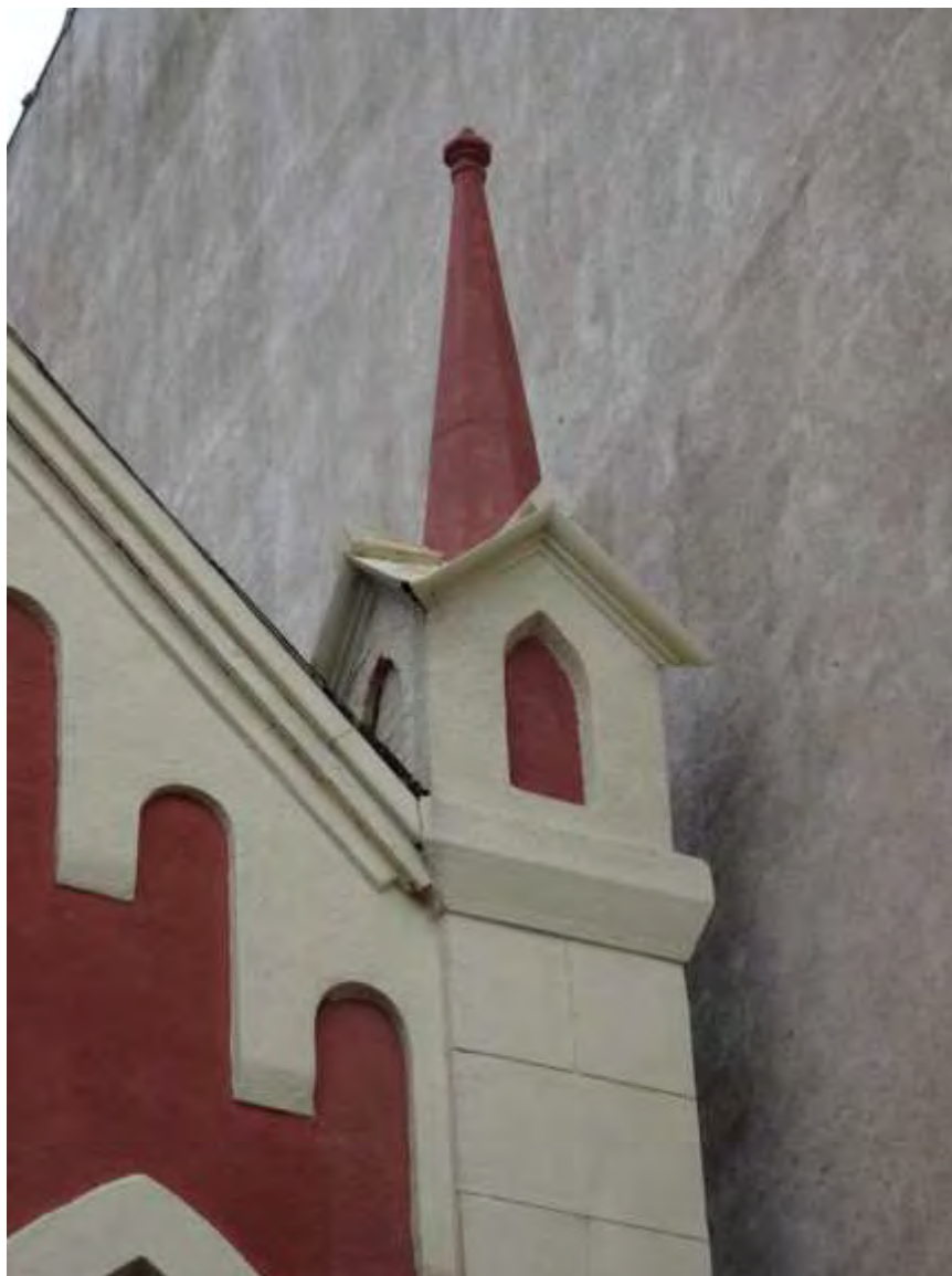
Photograph 2. Detail view of cross-gabled turrets with inset lancet panels and pinnacles flanking the property.
