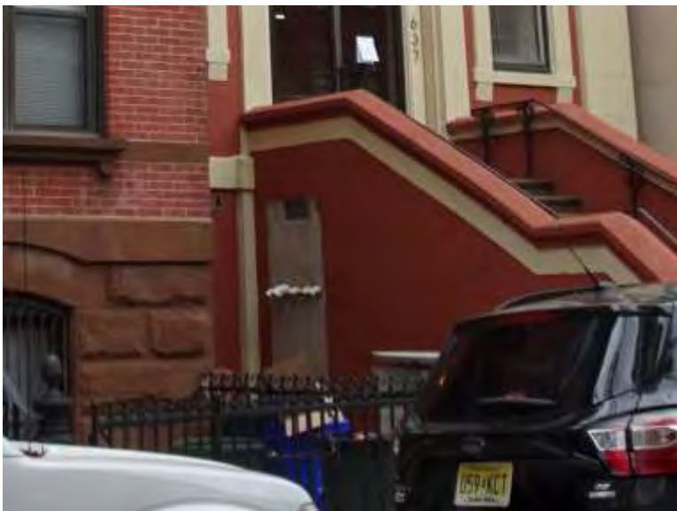
Photograph 7. Street-level modifications include infill of openings on the façade and introduction of utilities on the stoop.
