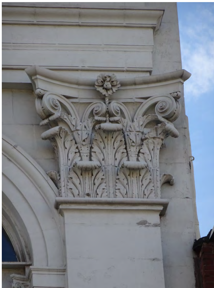
Photograph 7. Detail view of the ca. 1915 terra cotta Corinthian pilaster capital on the primary elevation of the building.
