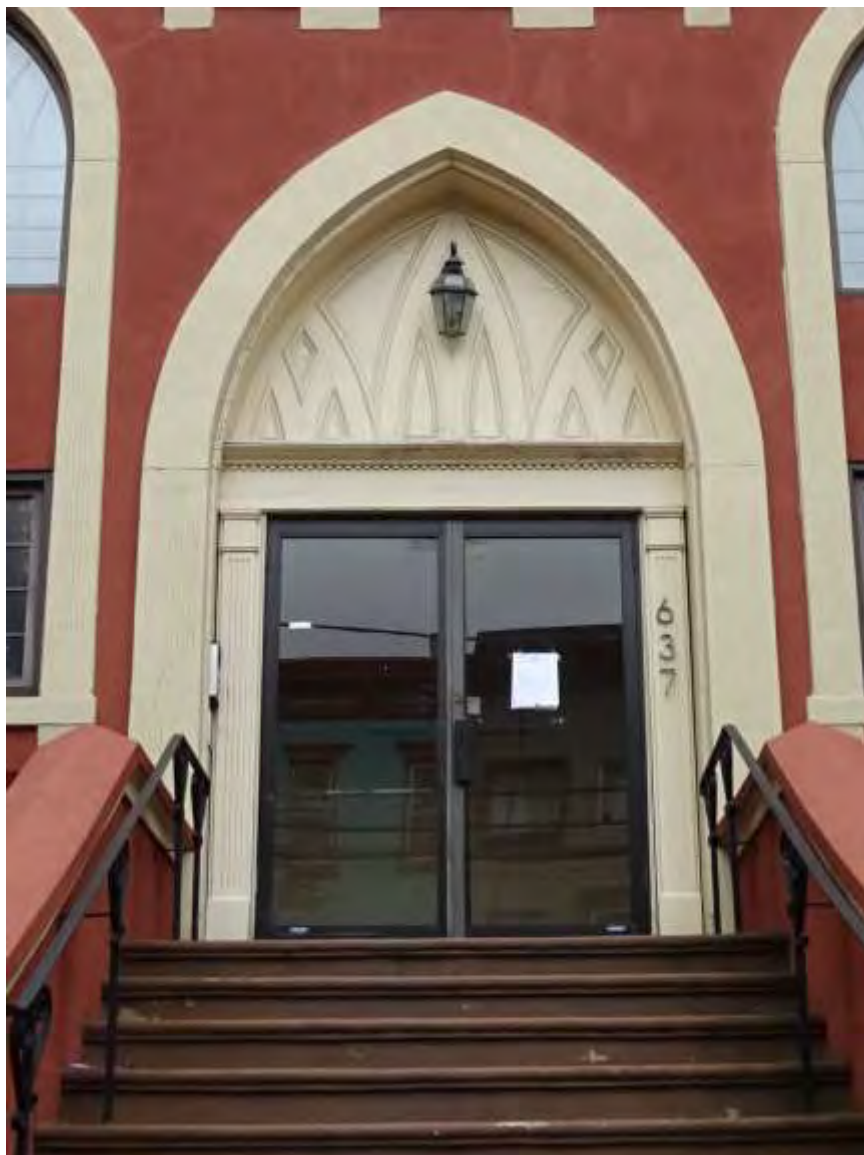
Photograph 4. View of main entry, with replacement doors set into original opening with intact wood tracery and fluted pilasters.
