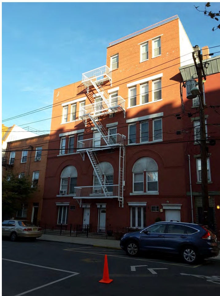
Photograph 10. View of the rear (west) elevation of Odd Fellows Hall / Lining Store building along Bloomfield Street.
