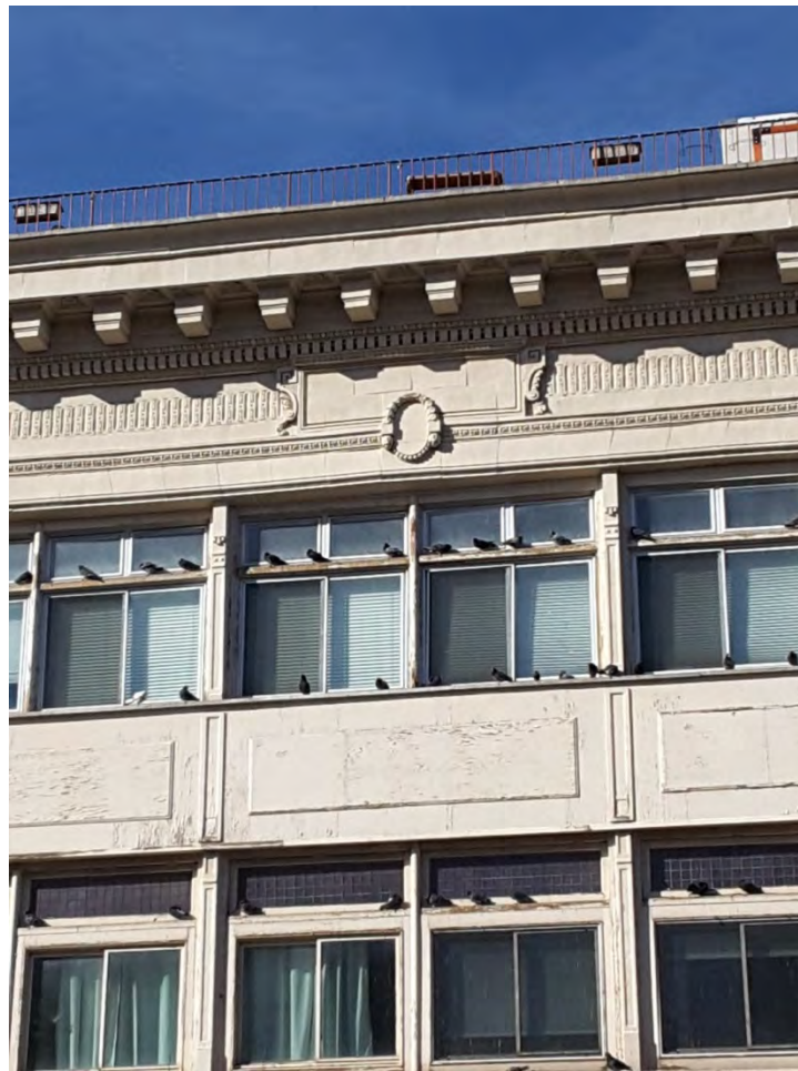
Photograph 3. Detail view of terra cotta ornamentation on the Washington Street façade of the Geismar-Meyer Co. Department Store building. Note the historicized ca. 1984 plywood panels below the third floor windows.
