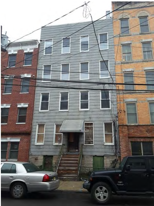
Photograph 3. 410 Monroe Street, view looking west.
