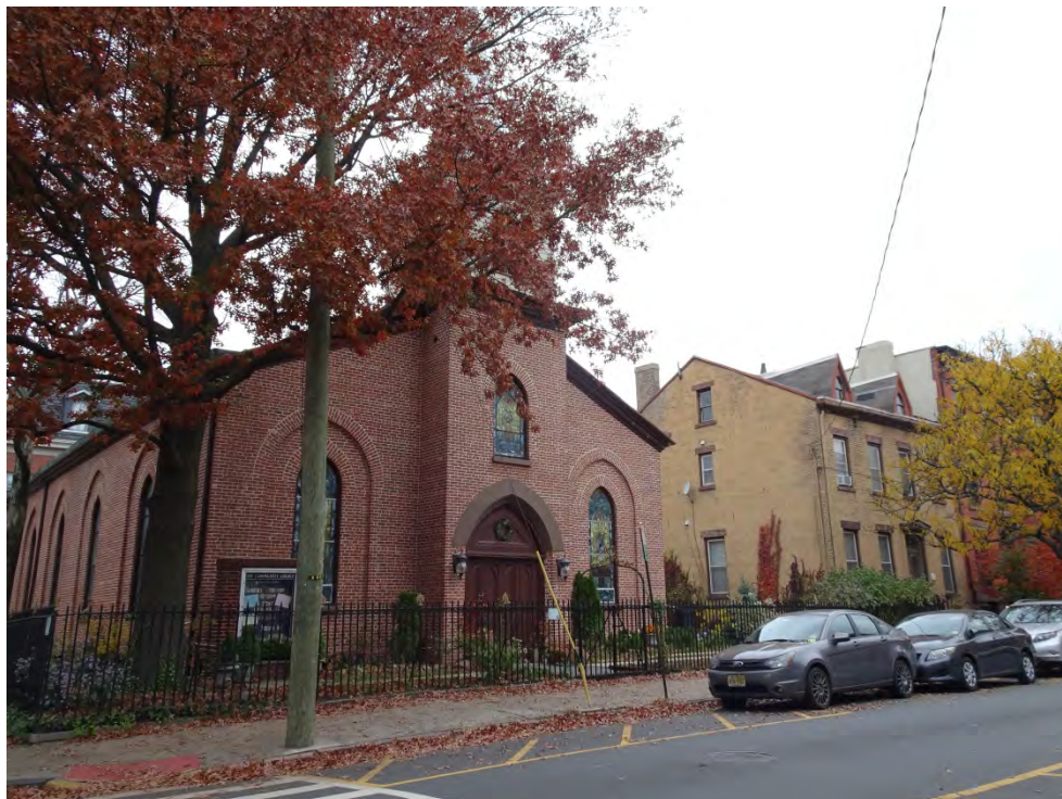
Photograph 1. Overview view of 600-606 Garden Street showing the Community Church of God and the rectory building, view northwest.
