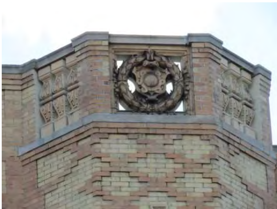
Photograph 3. Detail view of the ornate parapet, view west.
