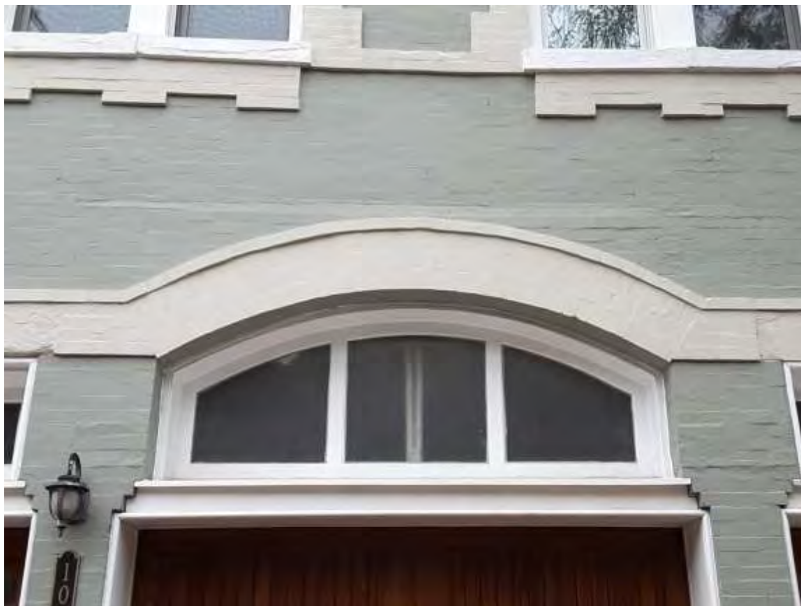
Photograph 2. Detail view of brick detailing on the façade and fenestration surrounds.
