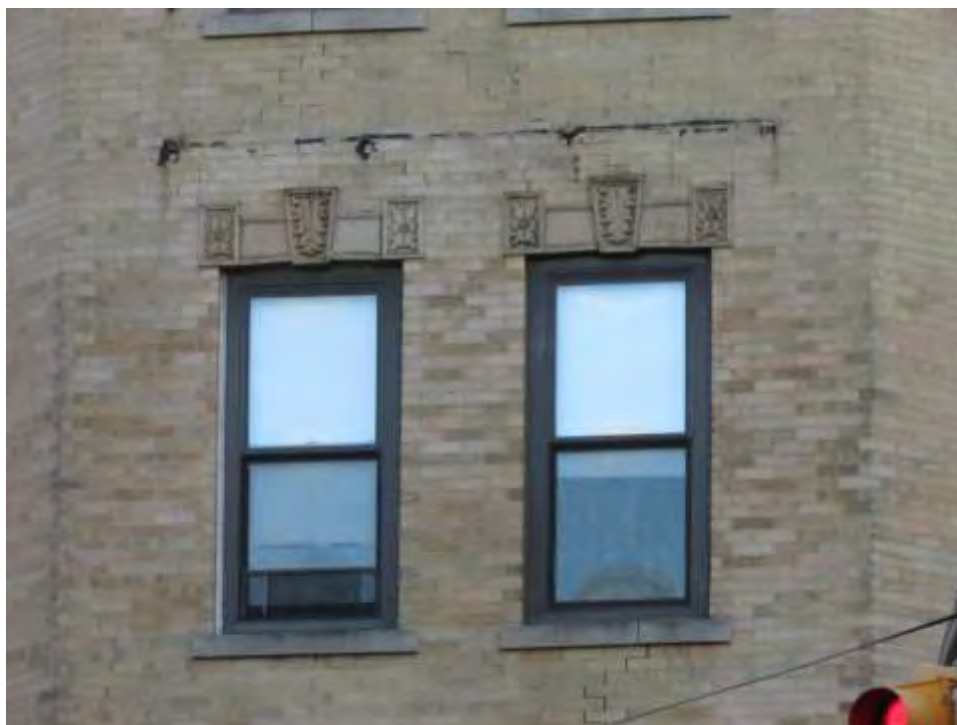
Photograph 7. Detail view of windows on a middle floor, view east.
