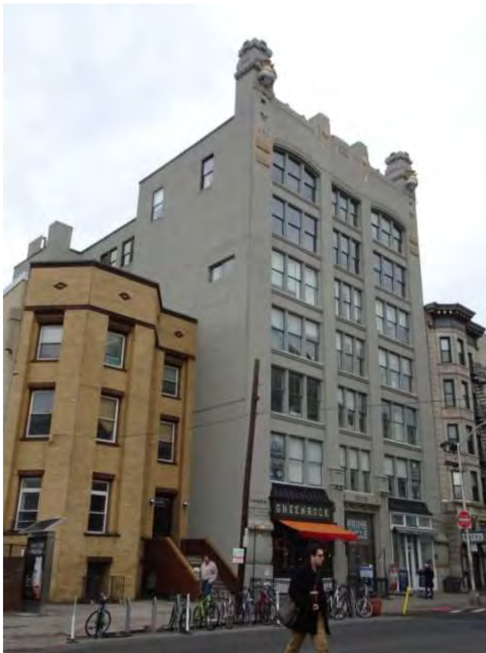
Photograph 2. Perspective view of the side (south) elevation, demonstrating the elevated ends of the cornice, looking northwest.
