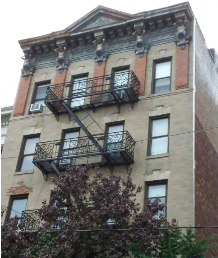
Photograph 2. Detail view of façade and ornate cornice, view west.
