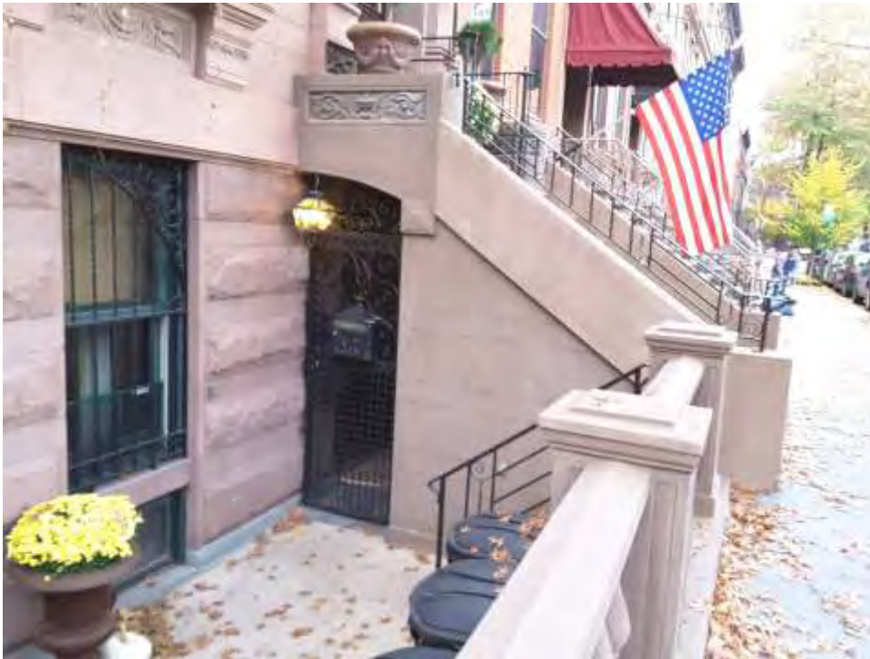
Photograph 6. Secondary entrance at the garden-level, view northwest.
