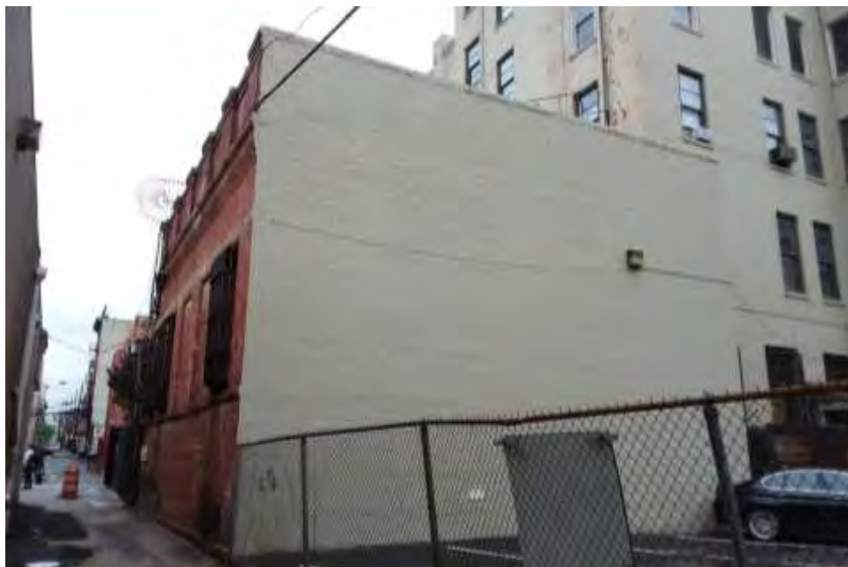
Photograph 6. A one-and-a-half-story rear annex is located on Court Street. View northeast.
