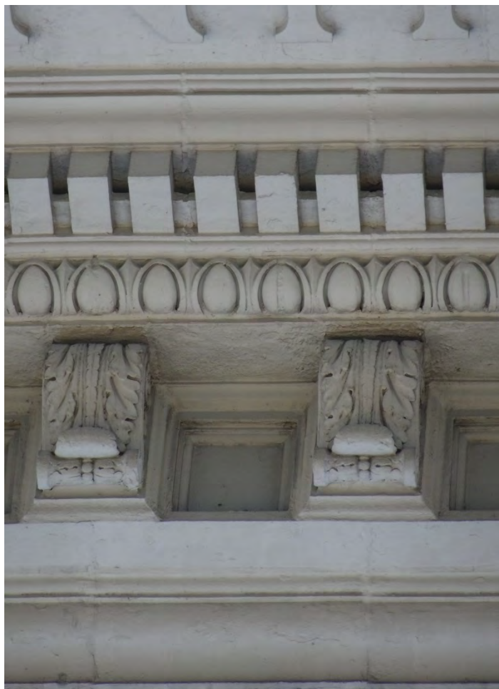
Photograph 8. Detail view of the historic terra cotta cornice ornamentation on the primary elevation of the building.
