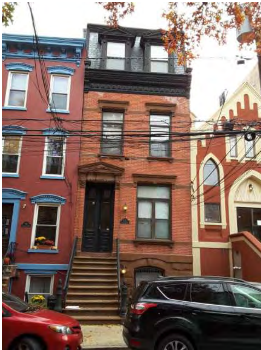
Photograph 8. Front elevation of the former Harry H. Hankins Residence at 639 Garden Street, which has been part of the former Temple Adath Emuno property since 1944. View east.
