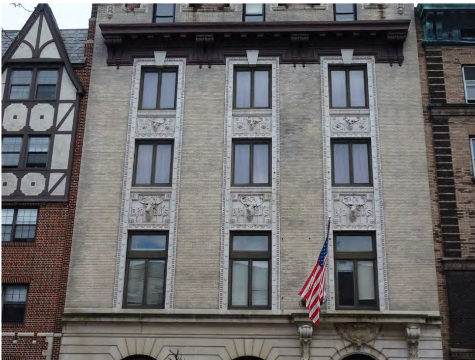
Photograph 4. Looking at the fenestration on the upper floors of the building, view east.
