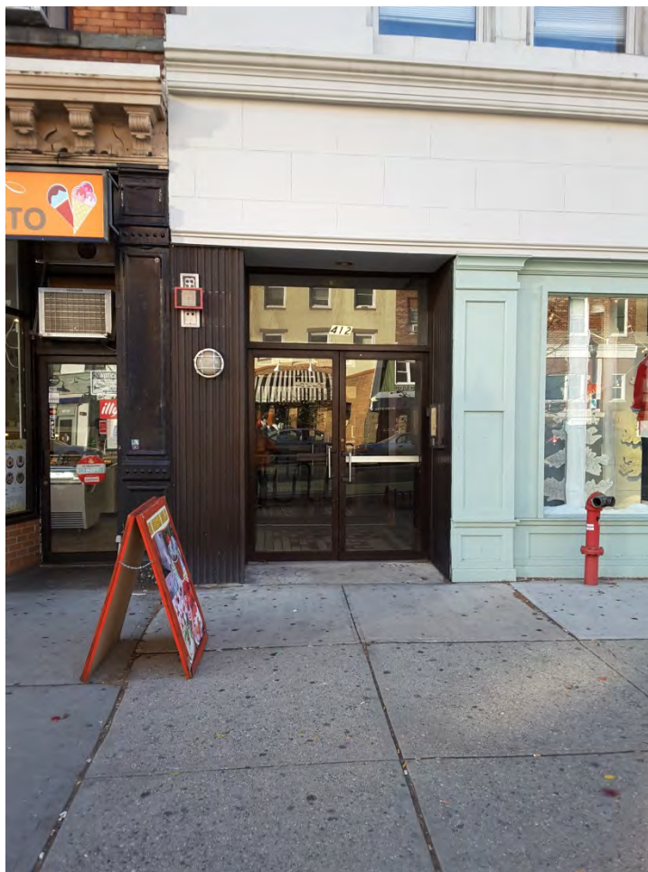
Photograph 4. View of the primary entry to the upper floors of the building from Washington Street.
