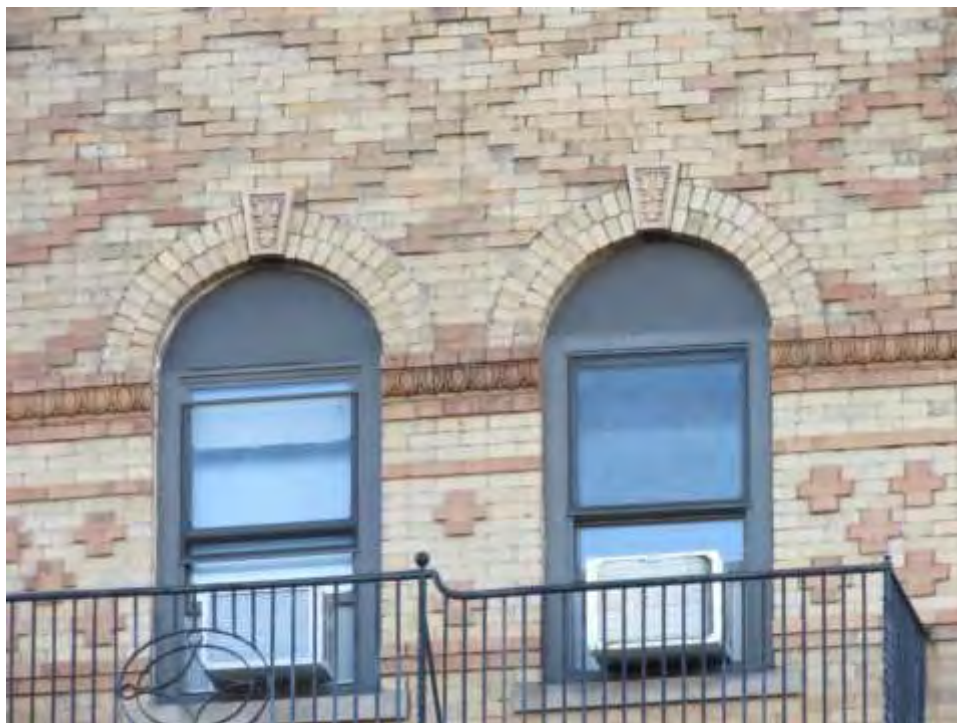
Photograph 6. Detail view of windows at the fifth floor, view west.
