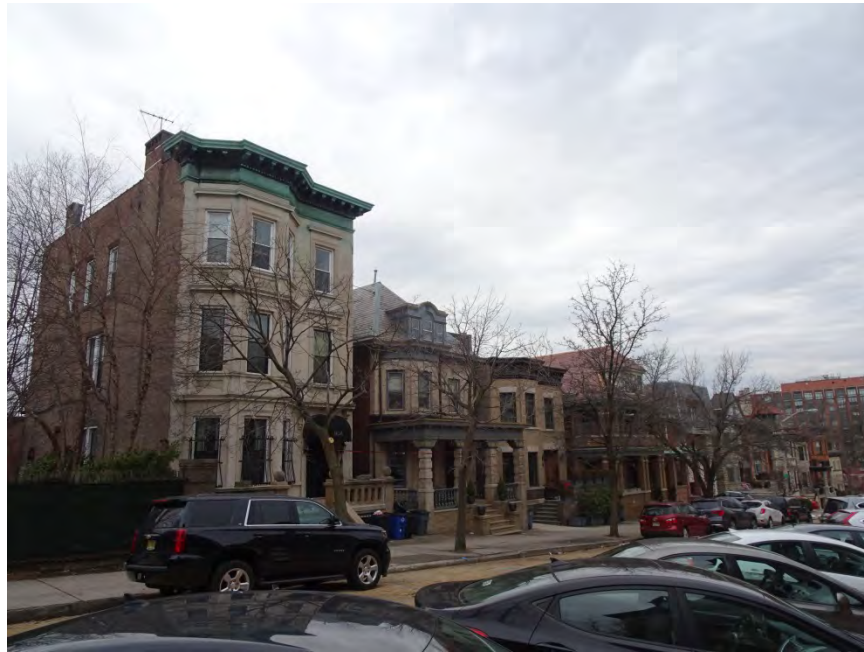
Photograph 7. View northwest along the 900 block of Castle Point Terrace.
