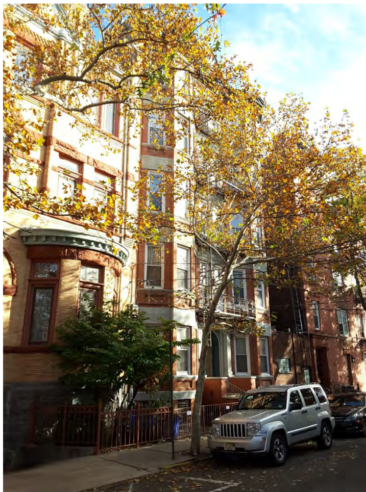
Photograph 2. View of the primary (south) elevation of the Marguerite apartment building at 106 11th Street, looking east along 11th Street.
