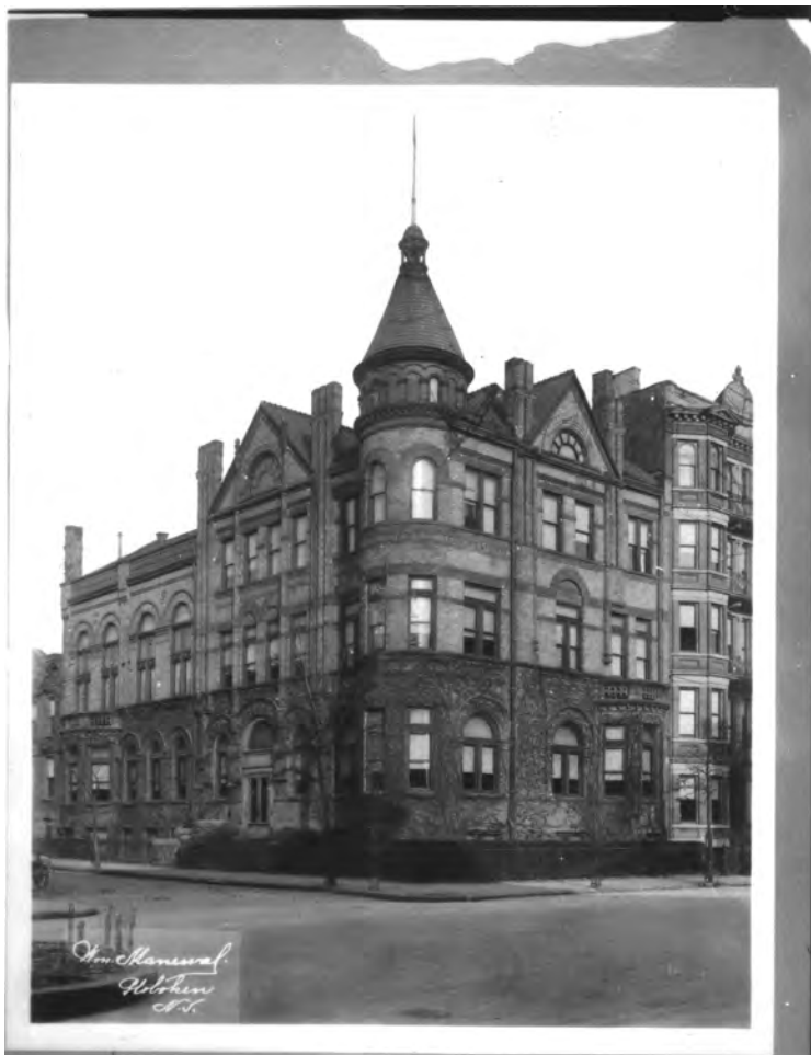
Figure 9. The apartments at 106 11th Street are visible in this ca. 1920 photograph of the Columbia Club building. Note the absence of the corner finials along the roofline (Source: Rutgers University).
