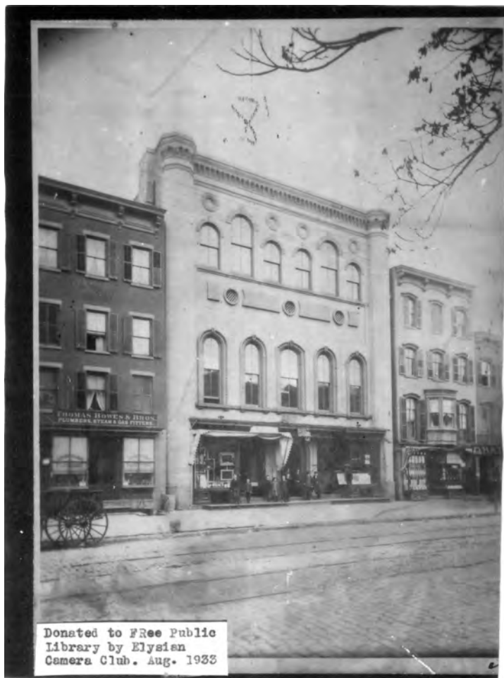
Figure 8. Photograph of Odd Fellows Hall ca. 1888 in the collection of the Hoboken Public Library, showing the third story added in 1881 (Source: Rutgers University).
