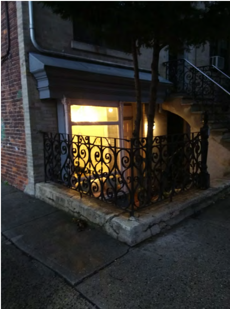
Photograph 4. Detail view of basement-level storefront, view northwest.
