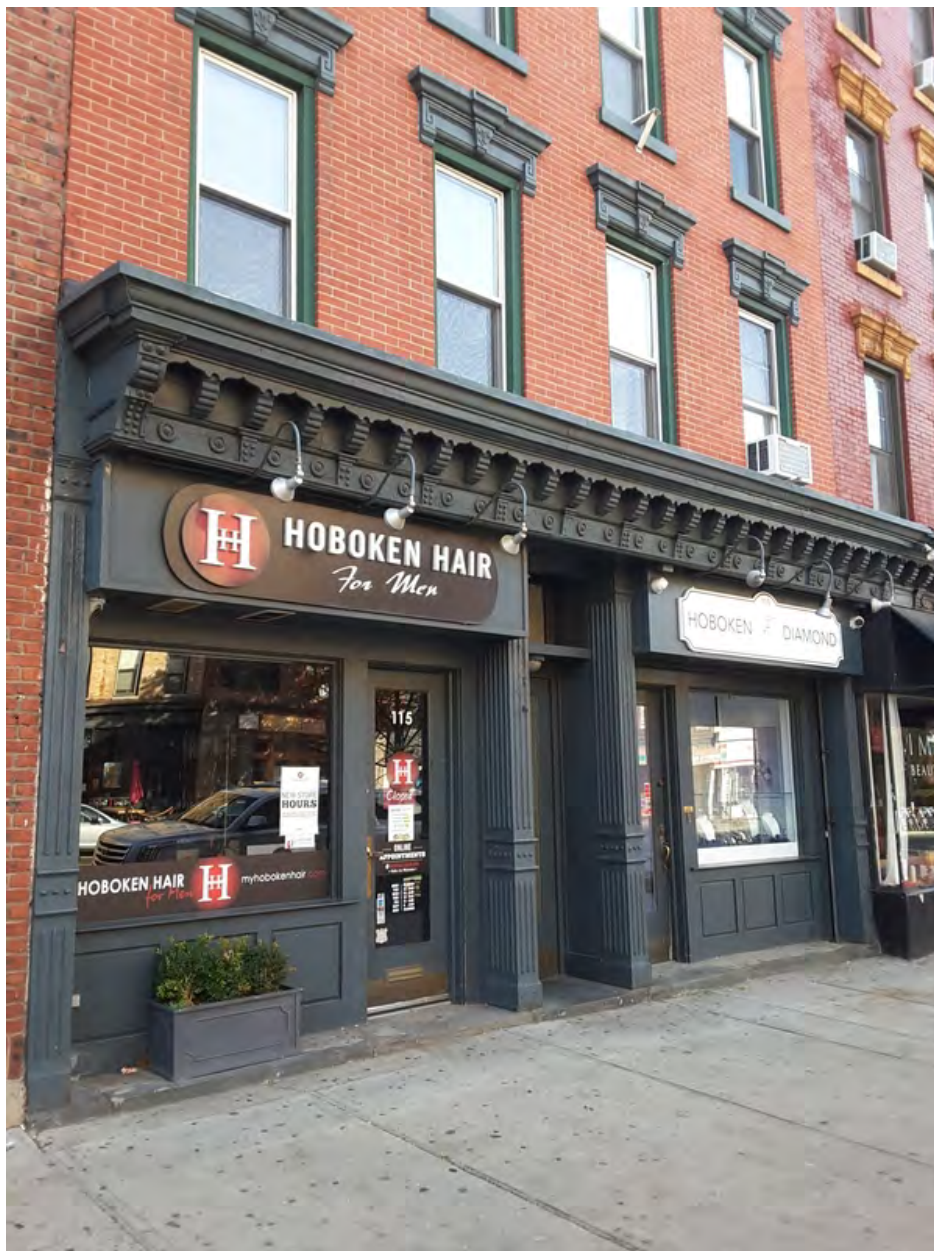
Photograph 5. Character-defining cast iron storefronts at 115 Washington Street. Note the decorative, projecting cornice, detailed pilasters, paneled accents, and separate entrances for public and private access.
