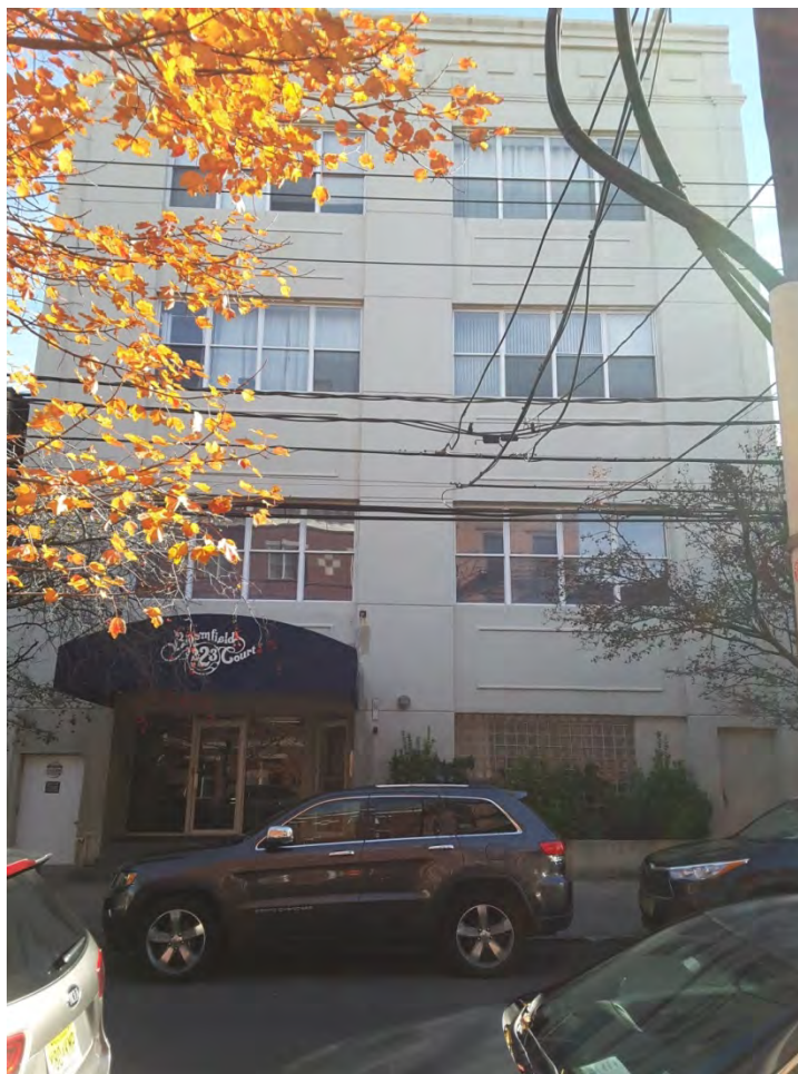
Photograph 6. The heavily altered Bloomfield Street (west) elevation of the Geismar-Meyer Co. Department Store building, showing access to the 232 Bloomfield Court units.
