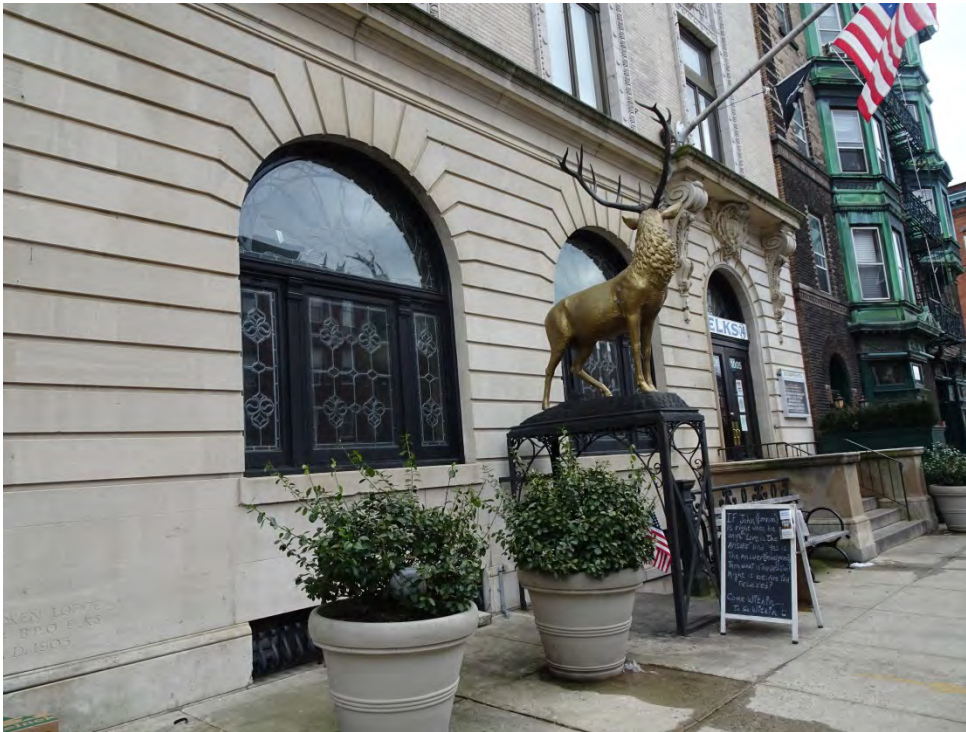
Photograph 3. Looking at the first floor fenestration, view southeast.
