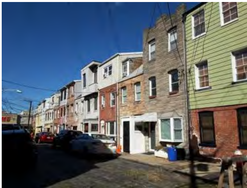
Photograph 5. View northwest of the north side of Willow Court North.
