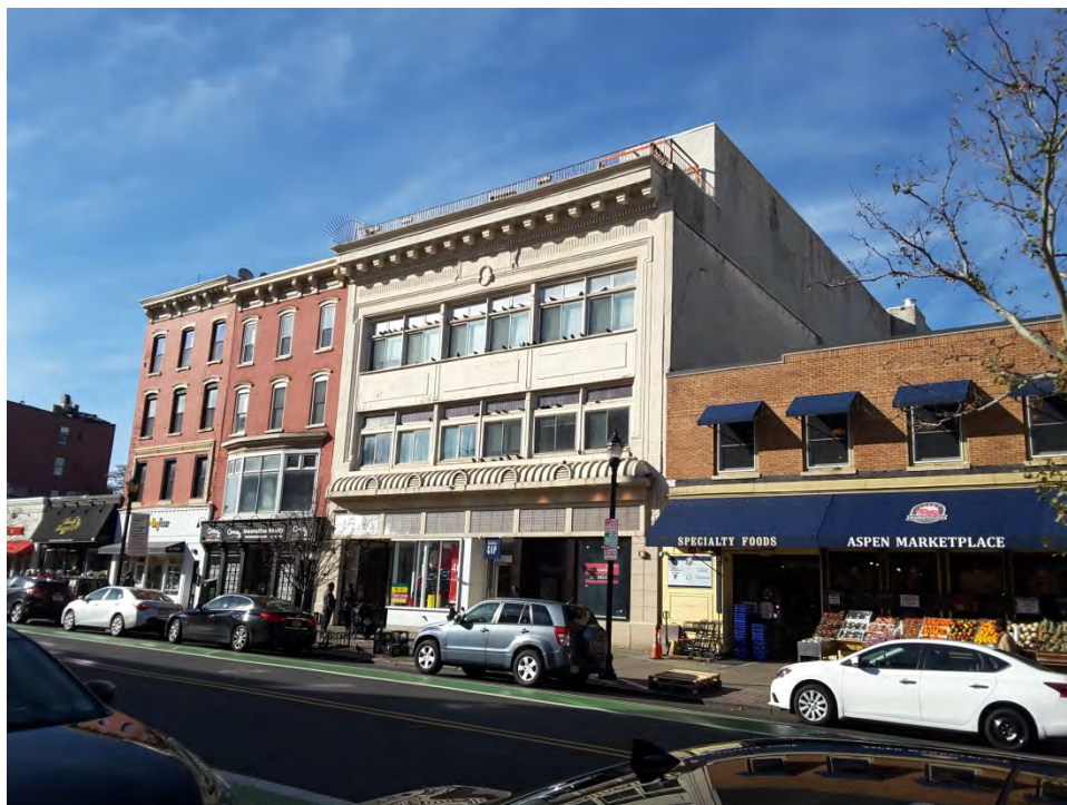
Photograph 2. View of the Geismar-Meyer Co. Department Store building in its setting on the commercial strip of Washington Street.
