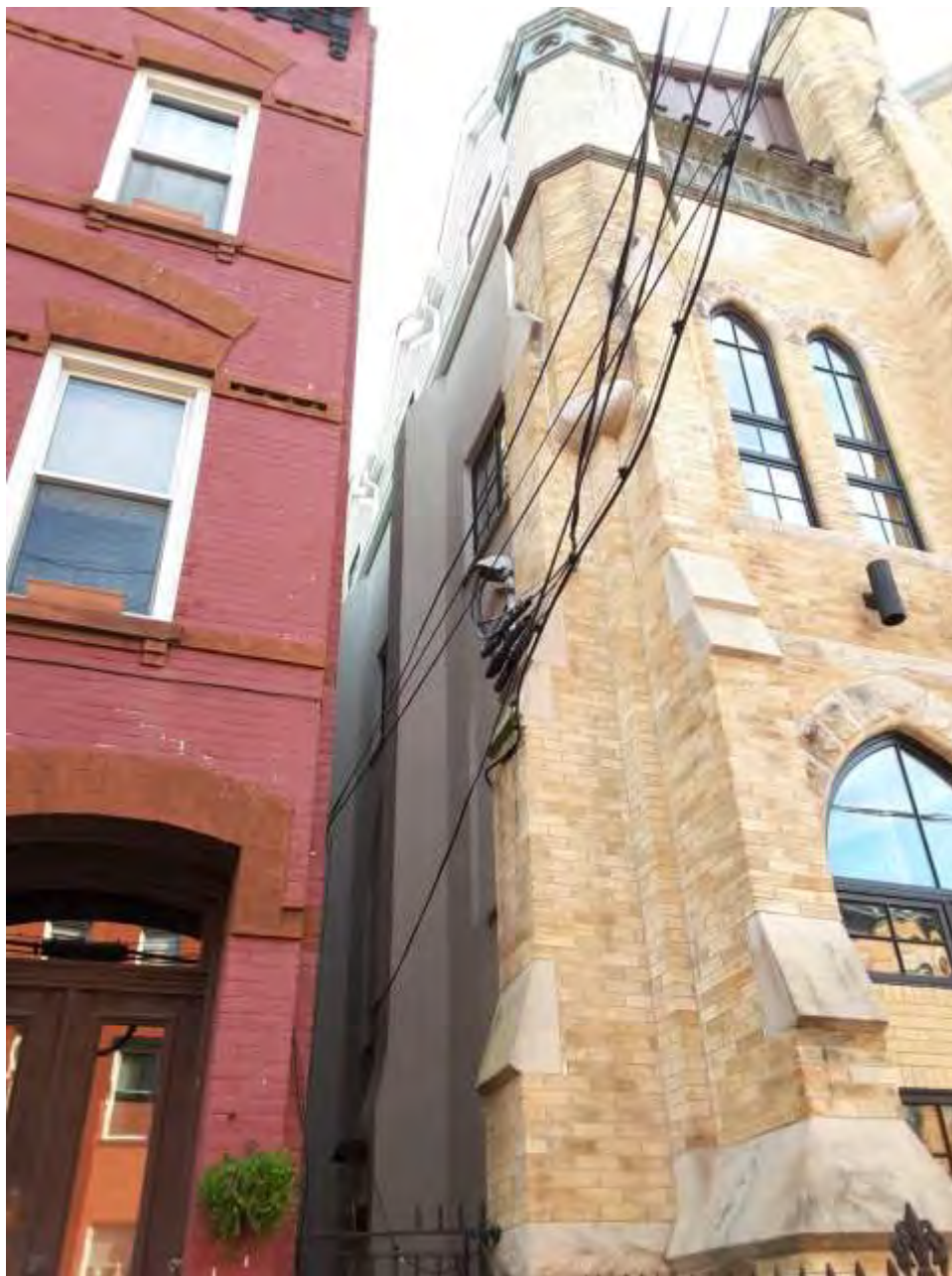
Photograph 6. Modifications to the side elevation during the 2011-2013 rehabilitation, view east.
