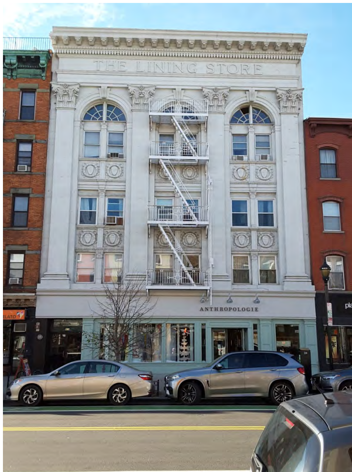
Photograph 1. View of the primary (east) elevation of Odd Fellows Hall / Lining Store building at 412 Washington Street.
