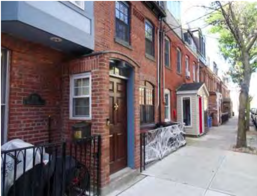
Photograph 9. View west along Seventh Street, near its intersection with Willow Avenue. Note the consistent rhythm of projecting vestibules along the streetscape and the ribbons of sawtooth brick above some of the second floor window openings.
