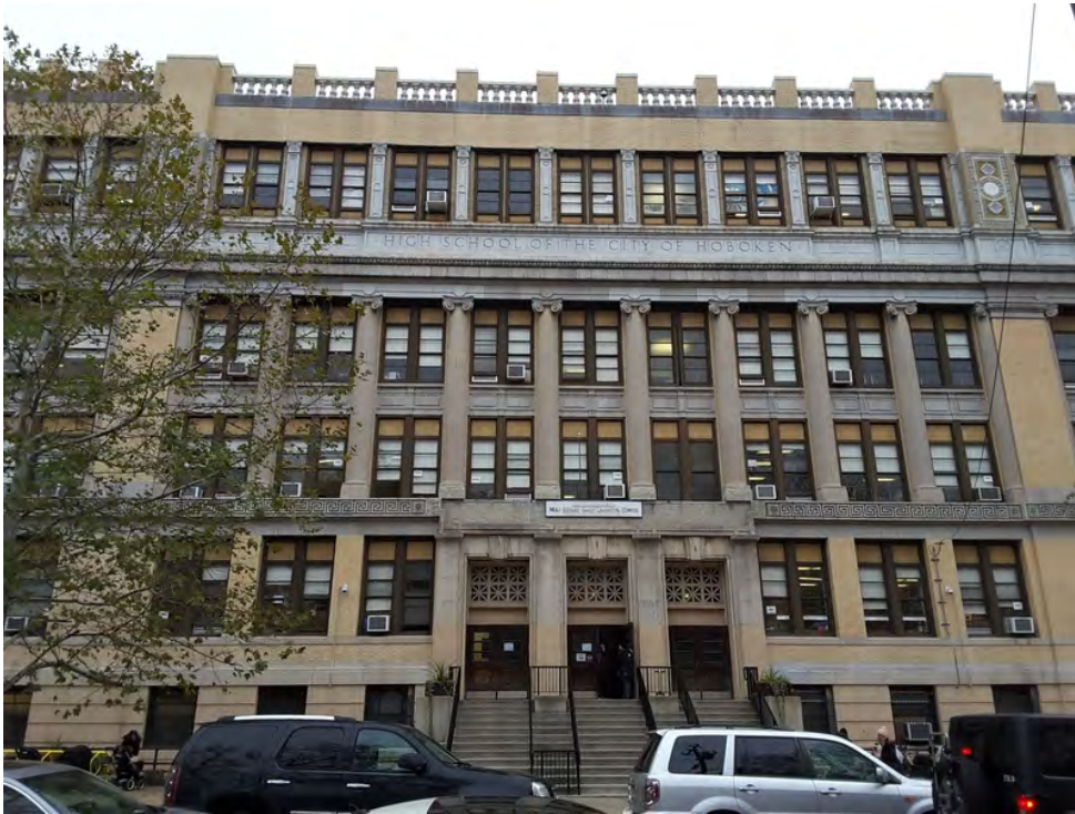
Photograph 2. Looking at the façade of the school along Garden Street, east.
