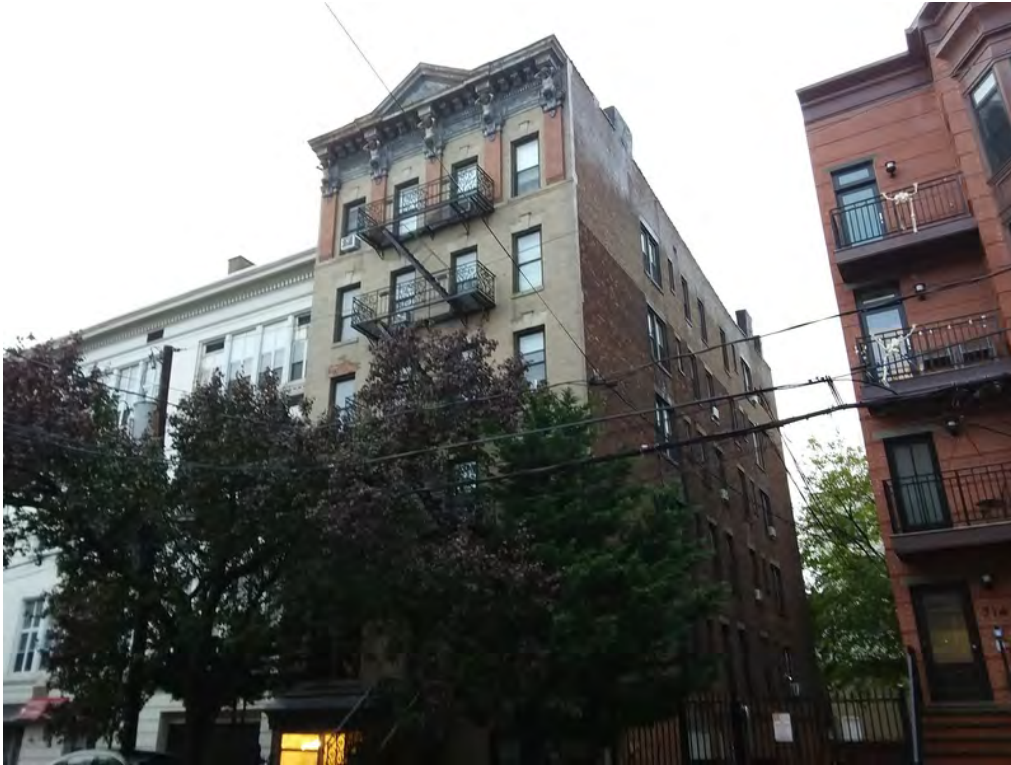
Photograph 1. Looking at the façade and north elevation of 710-712 Adams Street, view southwest.
