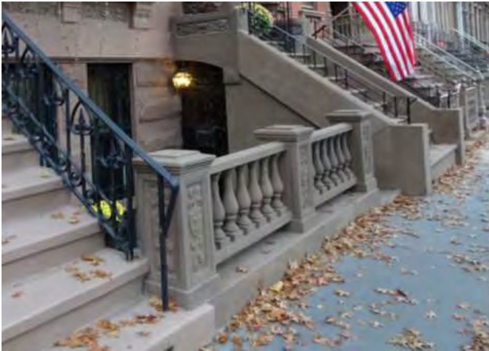
Photograph 4. Detail of the balustraded areaway at the Himpler Residence, view northwest.
