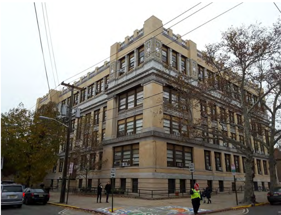
Photograph 3. Looking at the south and east elevations of the school building, view northwest.
