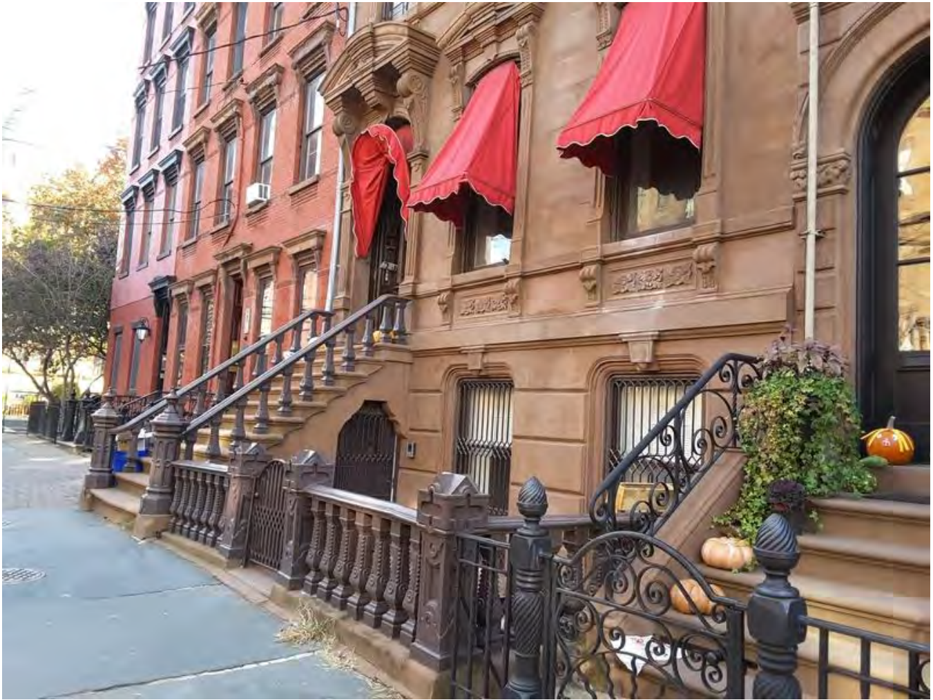
Photograph 3. Detail view of areaway fencing, stoop railings, and window and door surrounds, view northeast from sidewalk on Bloomfield Street.
