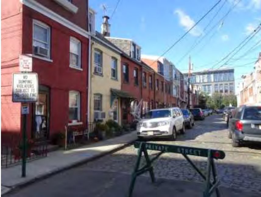
Photograph 1. View southwest of the south side of Willow Court South, from Willow Avenue. Note the surviving shared bracketed hoods at 3-5 Willow Court.
