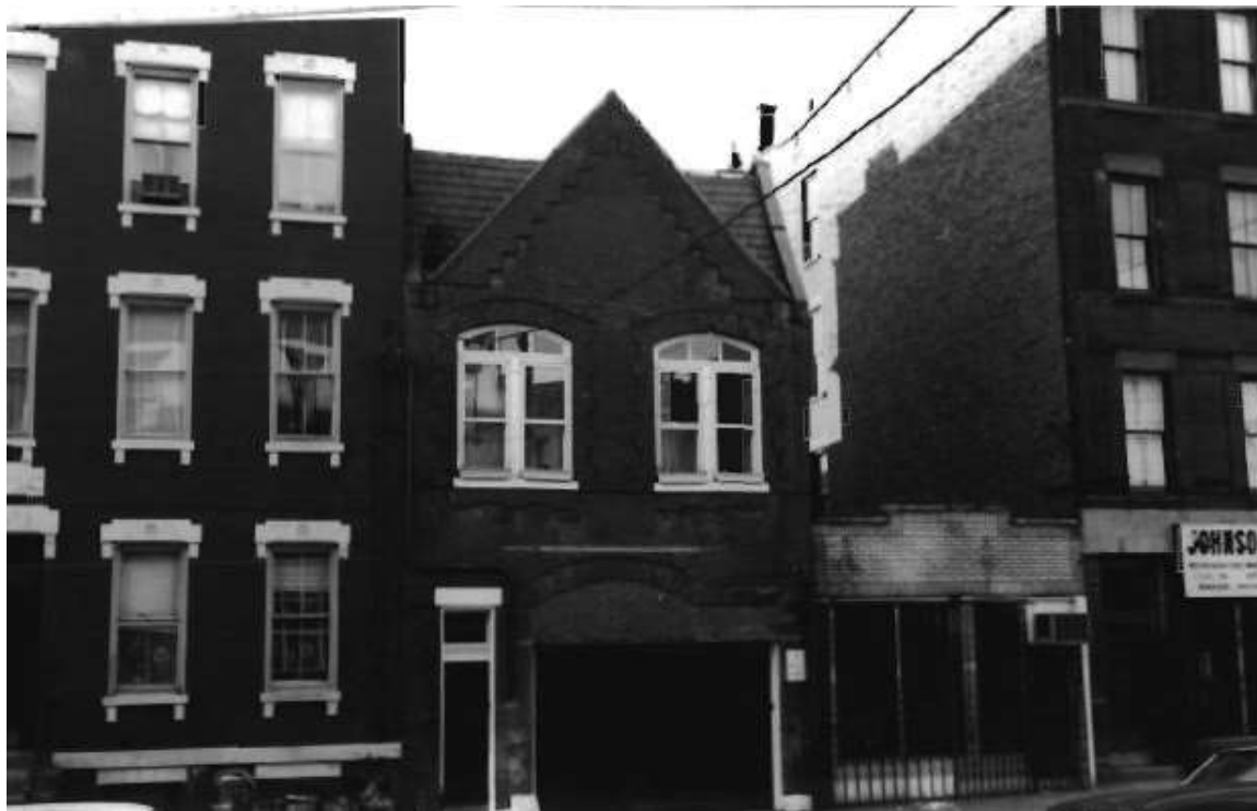
Figure 7. Documentation from the 1978 Hoboken New Jersey: A Physical and Social History, Vol. 5 . Note the evident character-defining features such as the steep parapet, corbelled details, and window surrounds (Source: NJ HPO).
