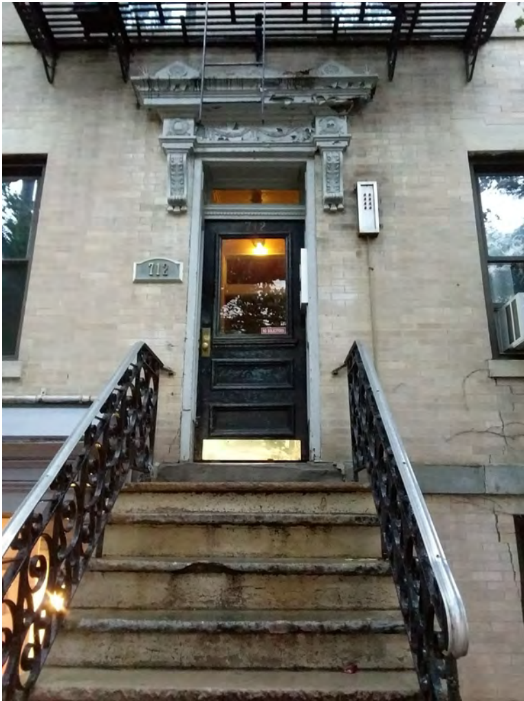
Photograph 3. Detail view of centered entryway on façade of building, view west.
