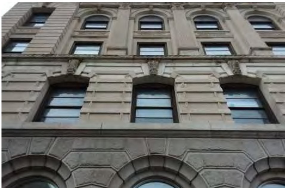
Photograph 2. Decorative stonework on the primary façade, view east.
