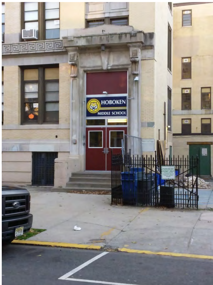
Photograph 6. Looking at the entrance on the east elevation of the building, view west.
