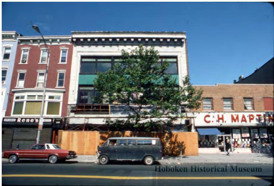
Figure 14. The Geismar-Meyer Co. building under renovation in 1984 (Source: Hoboken Historical Museum).
