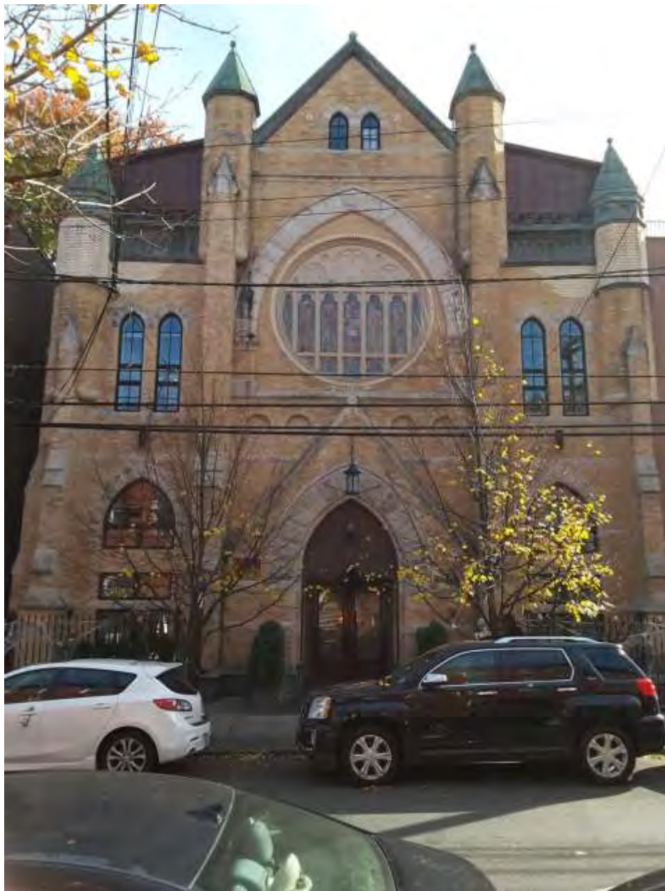
Photograph 1. Front façade of the Vestry at 829 Bloomfield Street, view east.
