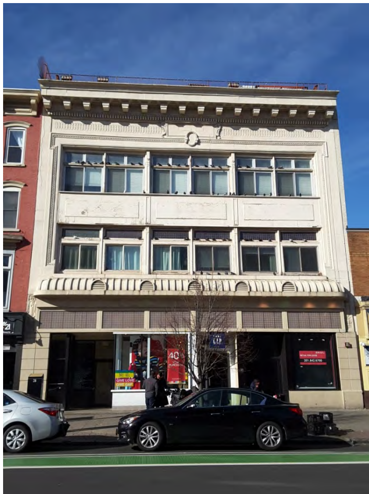
Photograph 1. The primary (east) elevation of the Geismar-Meyer Co. Department Store building on Washington Street.
