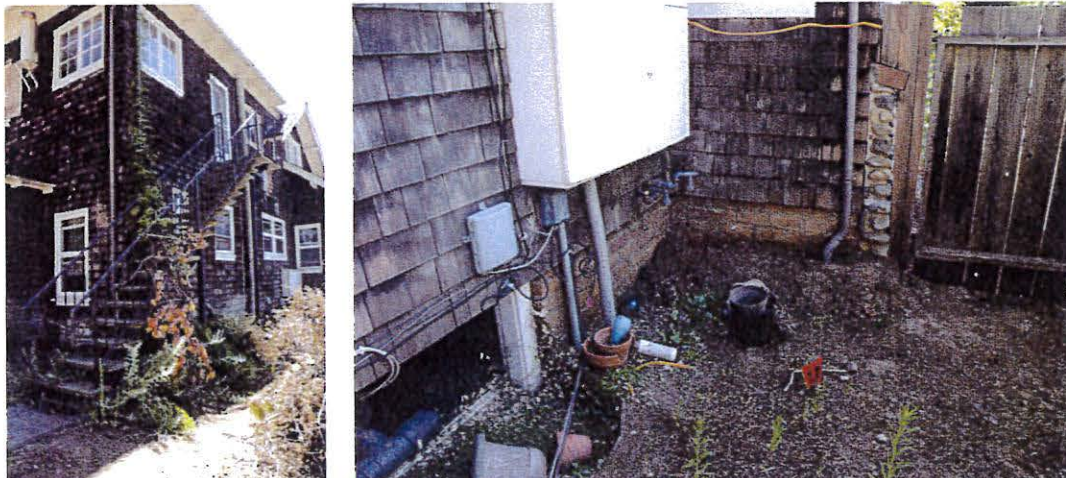
Image 13-14. Details of the North façade including the concrete plank stair with metal railings (left) and the corner of the stair projection with brick foundation, wood shingles and applied river rock base with brick sill course.
