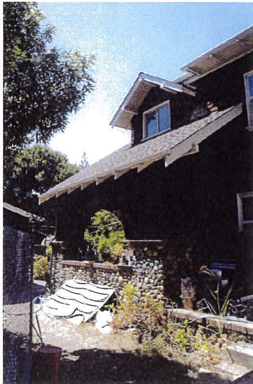
Image 17-21. South façade, the east end shown in the upper images and the west end at the bottom left image with a detail of the heavy pier and shingled arch of the covered entry at the bottom right.
