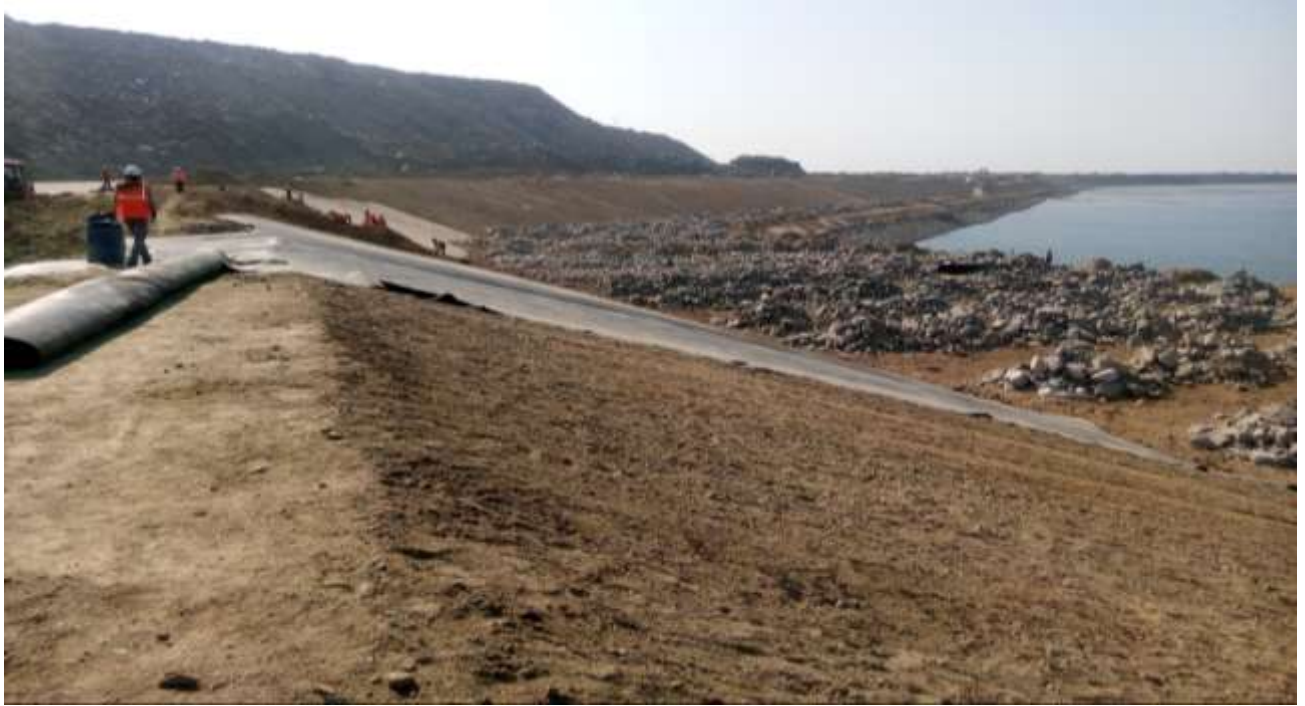
HDPE laying in tailing dam
