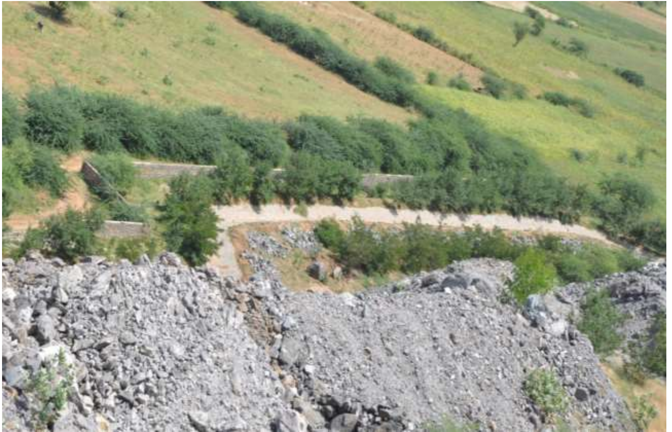
Garland Drain Photo
