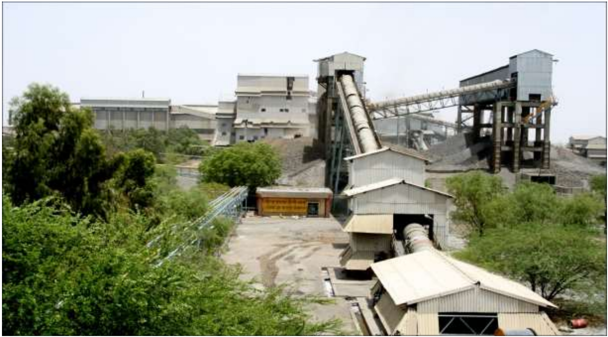
Covered conveyer belt
