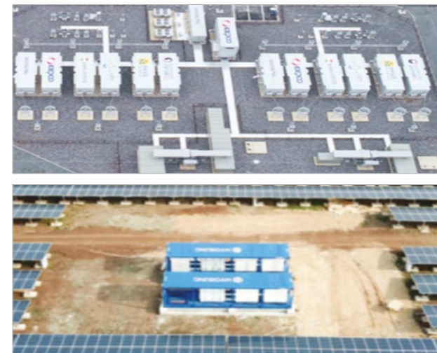
Figure 6 | Overall View of Containerized MV Station
