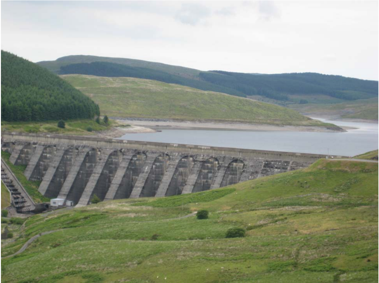
Figure 1.2. The Nant-y-Moch Dam in 2011 – No Symptoms of ASR after 50 Years – Constructed with Reactive Aggregate and 25% Fly Ash
