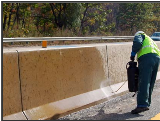
Figure 8.13. Photograph Showing Topical Application of 30%-LiNO 3 Solution to Concrete Pavement in Idaho
