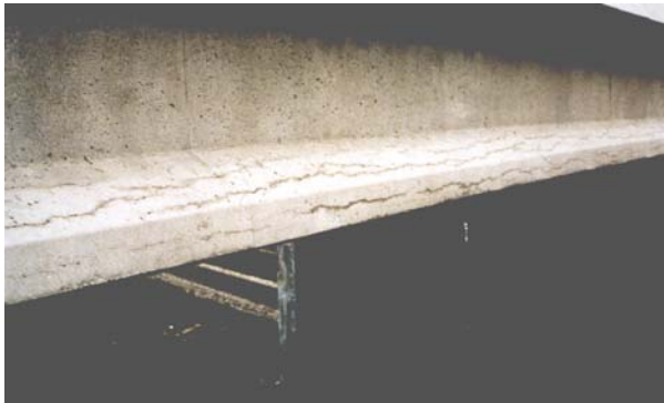
Figure 3.1. A. Map-cracking in the wing wall of a 30-year-old bridge structure affected by ASR (CSA 2000). B. Severe map-cracking and associated gel staining around cracks in a median highway barrier affected by ASR. C. Well-defined crack pattern associated with the development of ASR in highway pavement; the orientation of predominant cracks is longitudinal, while map- or pattern-cracking is also identified. D. Preferred alignment of cracks in an ASR-affected concrete column. E. Longitudinal cracking in a precast, reinforced concrete beam affected by ASR.
