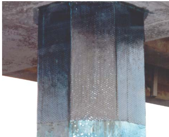
Figure 8.16. Photograph Showing Topical Bridge Column Wrapped with FRP (Carse 1996)
