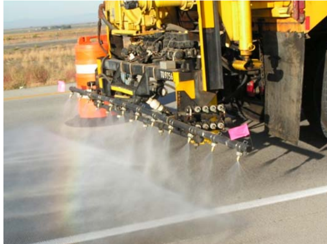
Figure 8.13. Photograph Showing Topical Application of 30%-LiNO 3 Solution to Concrete Pavement in Idaho
