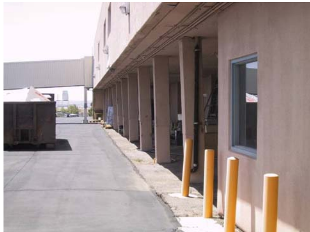
Figure 3.4. A. Relative movement of abutting sections of parapet wall in a bridge structure affected by ASR (Stark 1991). B-D. Expansion of concrete pavement due to ASR (overlaid with asphalt), which pushes against the adjacent building foundation causing shearing of concrete columns. E. Concrete sidewalk made with alkali-carbonate reactive limestone aggregate. Originally, the sidewalk and the curb were adjacent to each other; however, the expansion of the sidewalk created a gap that had to be filled with asphalt.
