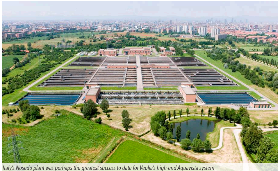
Italy’s Nosedo plant was perhaps the greatest success to date for Veolia’s high-end Aquavista system
