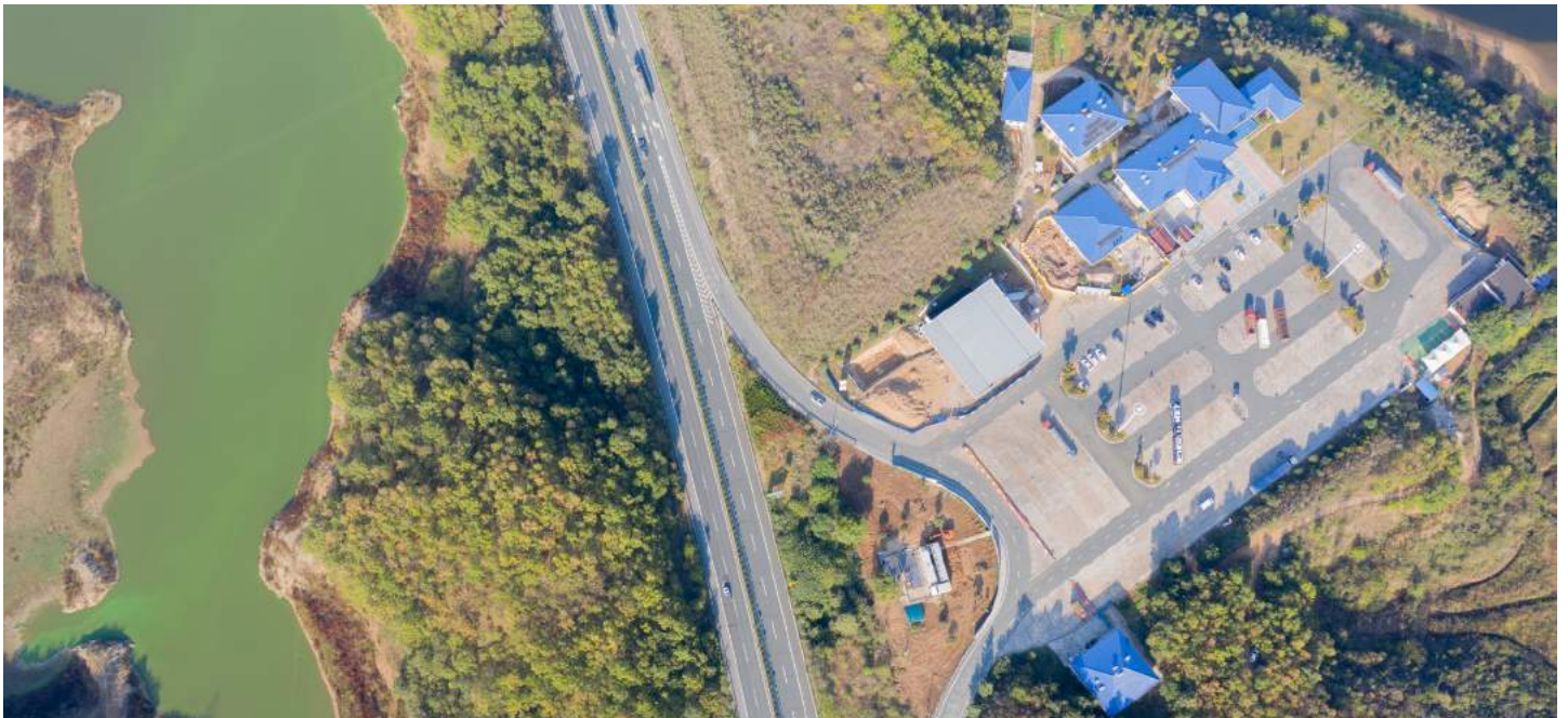
Fluence's decentralised modular units were the perfect solution for roadside installations in Hubei, China
