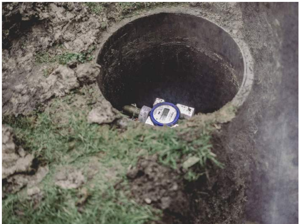
Kamstrup's smart meters with in-built acoustic leak detection helped enable the data-driven water revolution
