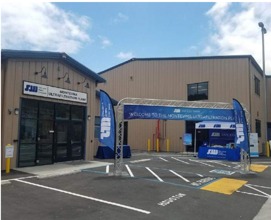
H2O Innovation's Montevina water treatment plant helps San Jose micromanage its seasonal water usage
