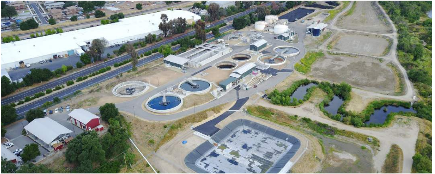
The super-flexible Paso Robles wastewater treatment plant can send water to the Salinas River when demand for recycled water is low
