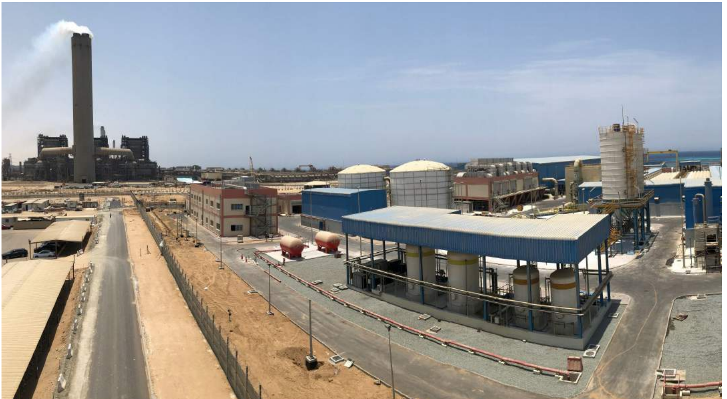
ACWA Power's work developing the second expansion to the Shoaiba 3 plant it owns marked the start of a renewed period of dominance in desalination PPPs
