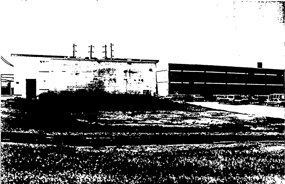
Final site restoration
