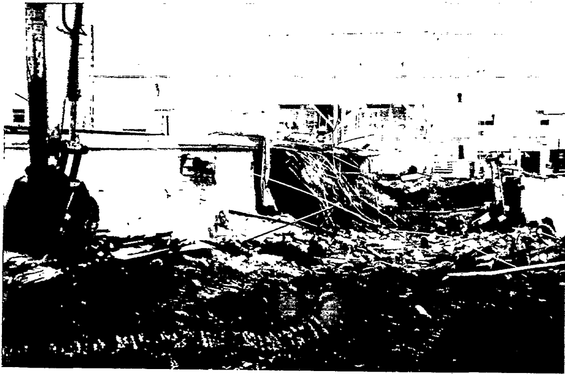
Demolition of pump room
