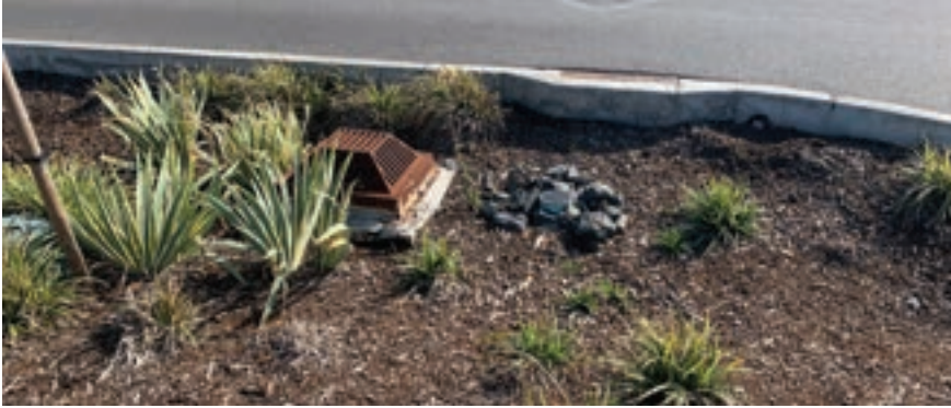
RAIN GARDEN MEDIANS SERVE AS CRUCIAL BASINS FOR STORMWATER
