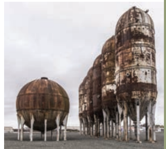
Acid ball & digesters
