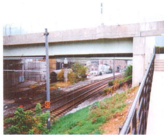
View of Light Rail Tracks
