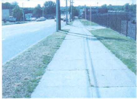
Section A. Sidewalk and electrical poles.
