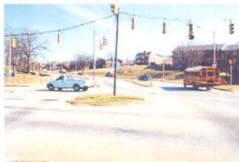
Looking north on Loch Raven to where southbound lanes split into two sections.
