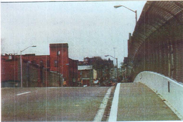
Monroe Bridge over railroad tracks
