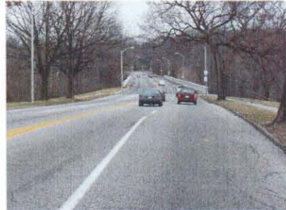
Bridge on Harford looking north.
