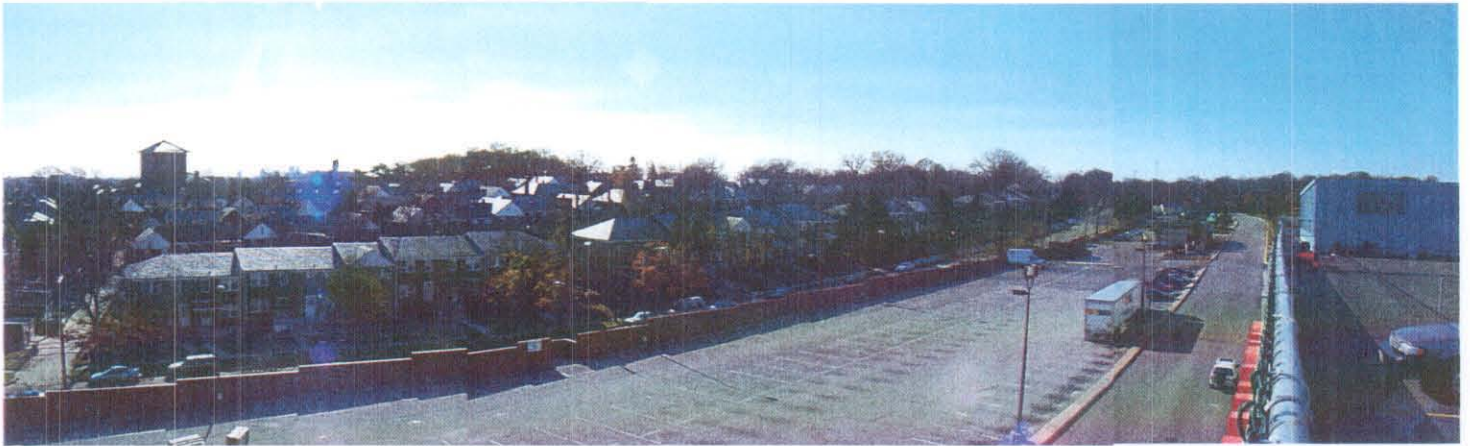
Looking west-southwest along existing driveway
