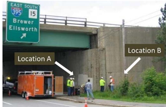
Figure 8.4. Photograph of bridge in Bangor, Maine. Location A is sheltered by the bridge deck, whereas Location B is exposed directly to precipitation. Sampling of concrete cores from each location showed strong correlation between moisture availability and ASR-induced expansion and cracking.
