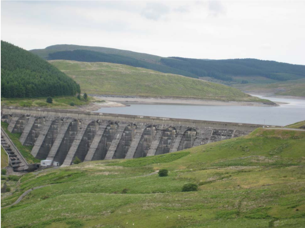
Figure 1.2. The Nant-y-Moch Dam in 2011 – No Symptoms of ASR after 50 Years – Constructed with Reactive Aggregate and 25% Fly Ash
