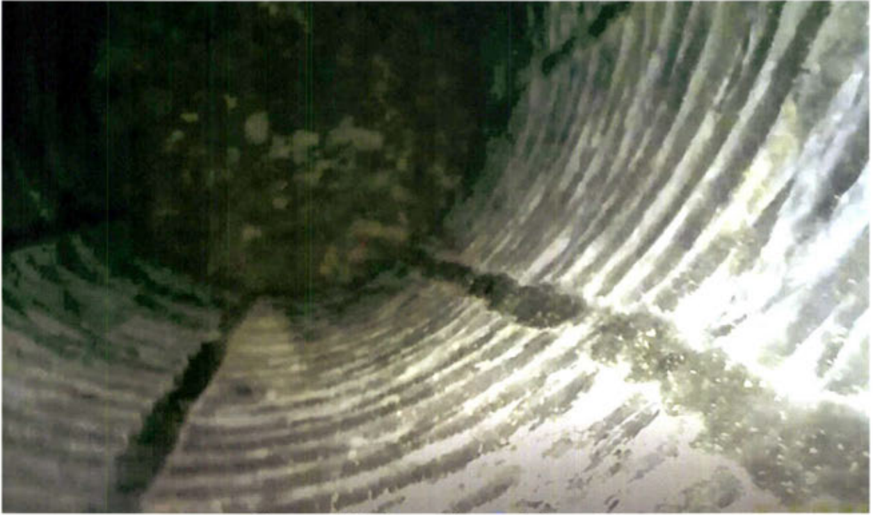
Closeup of the base of the core hole at -25'
