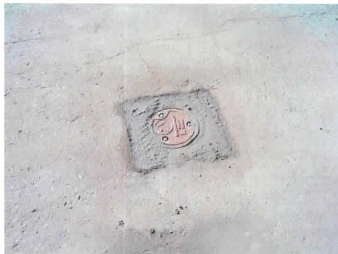
Photo 6. Groundwater Monitoring Well MW-4
