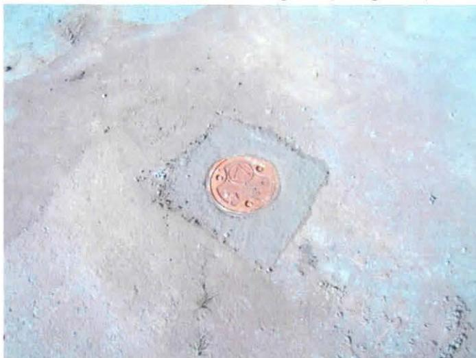
Photo 5. Groundwater Monitoring Well MW-3
