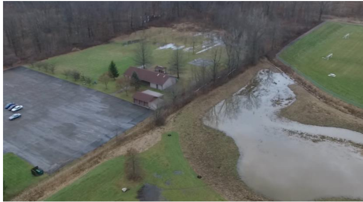
Figure 24: Aerial Image of Fairlawn Park, showing oxbow wetland and adjoining exposed and channelized stream corridor.
