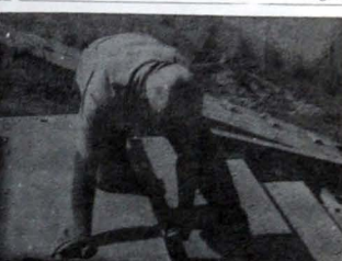
With construction now complete, new stairways will make access to the lower parking lots easier.
