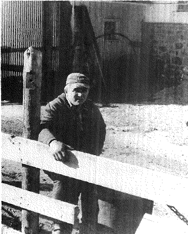
Donald Schultze, Rt. 1, Box 193, Bristol, stands at the fence line on the Russell Mott farm. Behind Schultze is the shed in which the well is located
