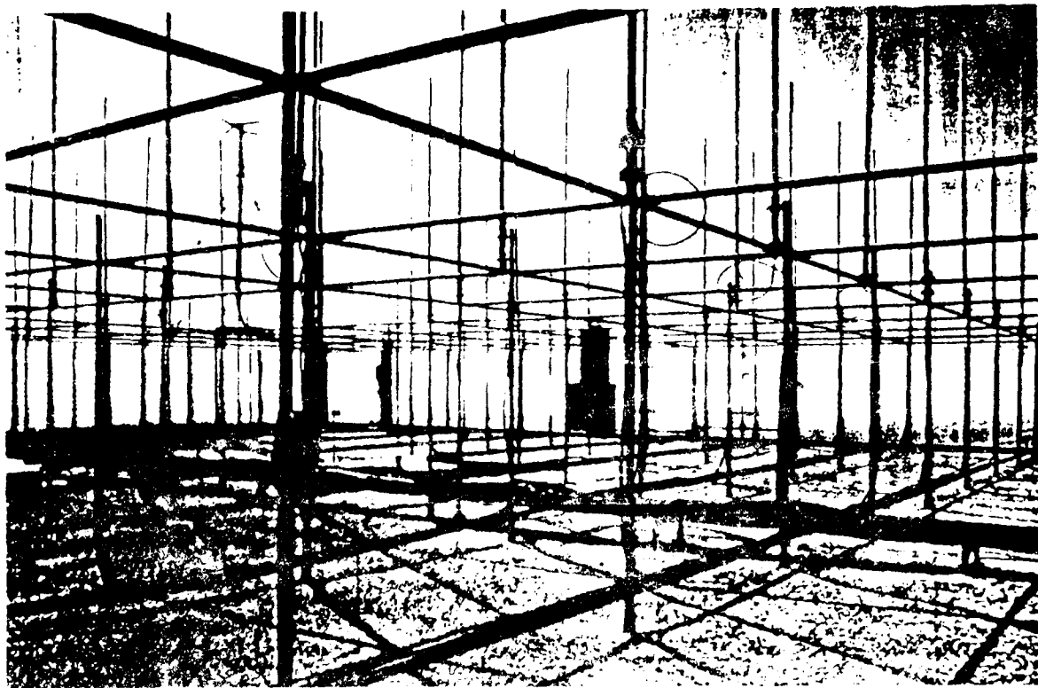
Figure 1 Land Mobile antennas on top of the Standard Oil Building in Chicago, Illinois.
