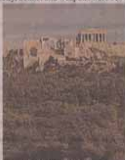
THE RECONSTRUCTED PARTHENON STILL DOMINATES THE ACROPOLIS IN ATHENS
