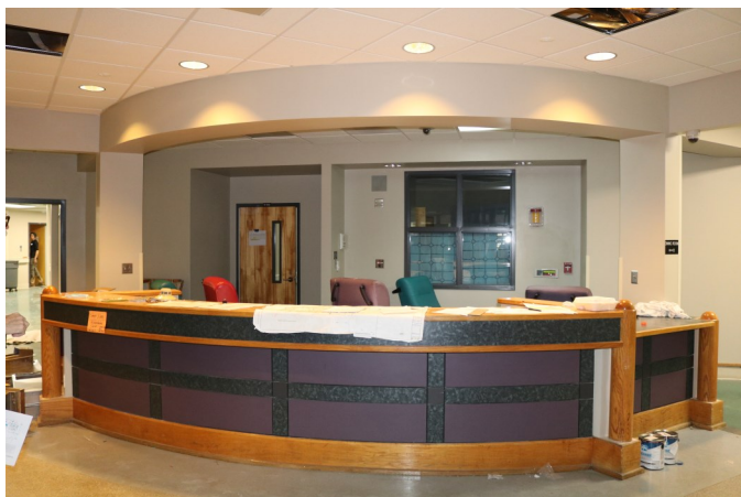
The reception area and nurses station of the new deaf unit. Story on pages 3
