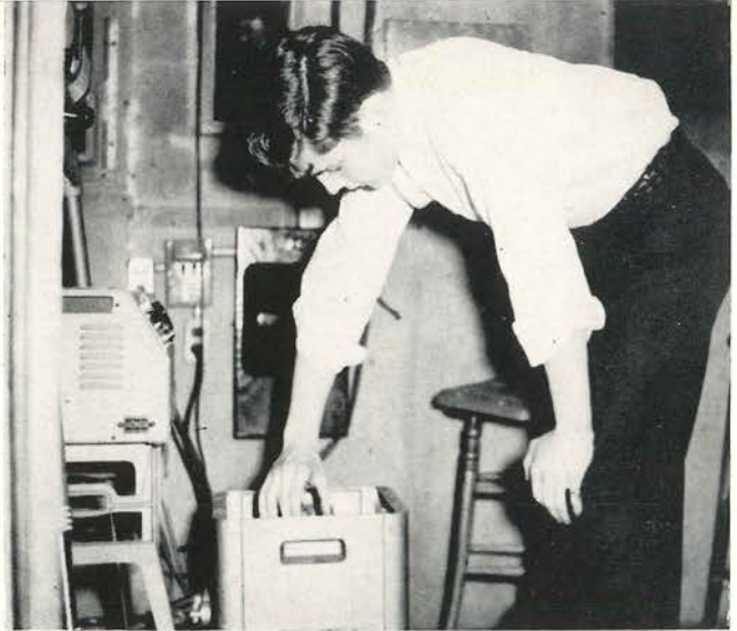
Bob Kirchgessner works busily behind the scenes in the electrician's booth during many assemblies and performances.
