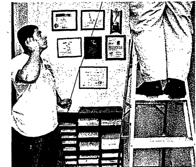
PC MD technician Tony Saucedo holds a fish tape while Leavitt pushes it through a wall at a Willowbrook CPA firm for The Unemployee. (Suzanne Tennant/Staff Photographer)
