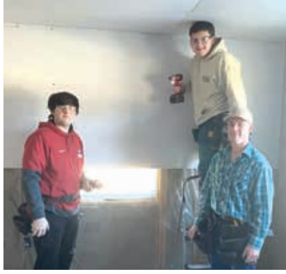
From left, DCTC students Andrew Mettler, Andrew Hartshorn and Weston Piper take a picture break screwing in the last screws on a sheet of drywall.
