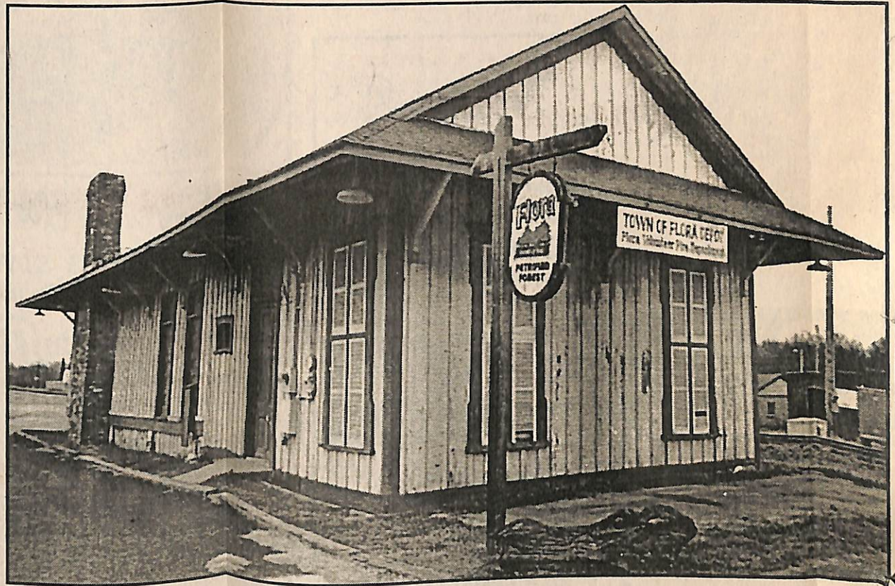
Flora railroad depot, recently added to the National Register of Historic Places, will be renovated
