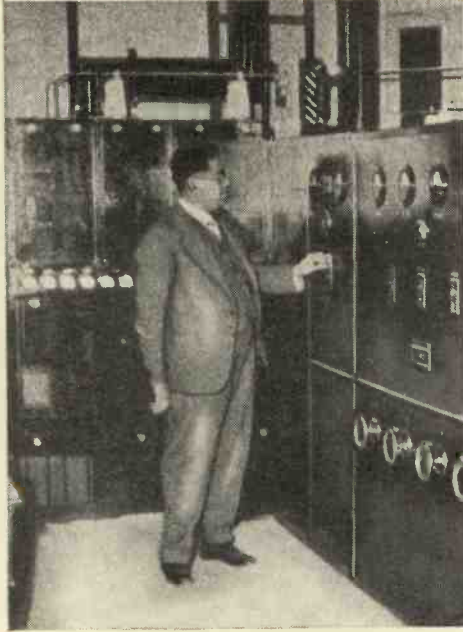
Left: The amplifier and control room.
