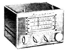
KARADIO MODEL 80-C, 3-band mobile receiver for underdash mounting. Covers broadcast band 540–1650 KC; 2.8–7.5 MC; 4.8–17.5 MC; which includes the 75 and 20 meter bands. 6 tubes: 6BA6 R.F., 6BE6 Mixer, 6BA6 I.F., 6AT6 demod.— 1st Audio, 6AQ5 output, 6X5GT rectifier.
