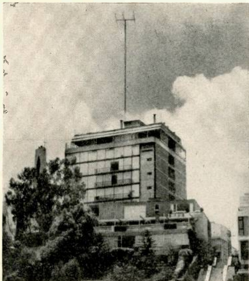
The tower atop this 10-story office building on the outskirts of Mexico City supports the beam antenna of XE1NE. It's no wonder that XE1NE can say that he has one of the highest ham radio antennas in all of the world—especially since Mexico City is about 7500 feet above sea level to start with.
