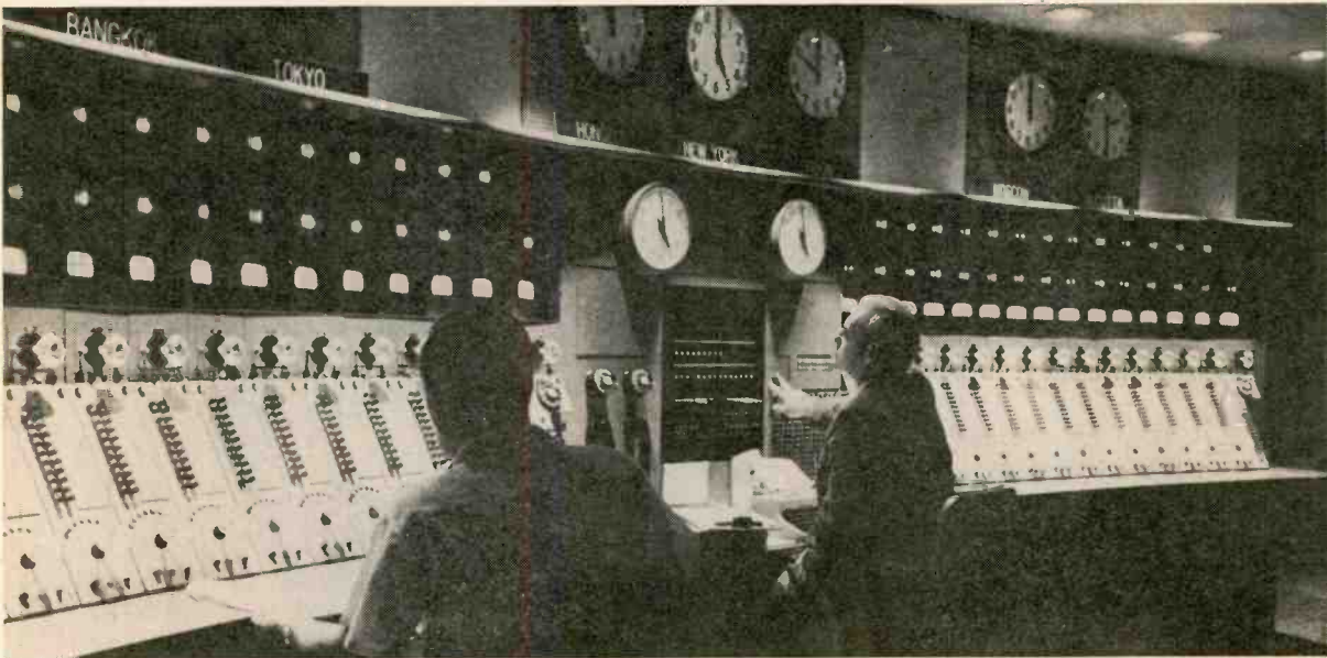
No one questions that short-wave broadcasting is used to disseminate truth and propaganda throughout the world. It is principally a contest between Radio Moscow and the Voice of America, and the latter now seems to have the upper hand. This is the master control of the VOA in its Washington, D.C., studios. Twenty-six programs can be fed simultaneously through this board to VOA transmitters here and overseas.
