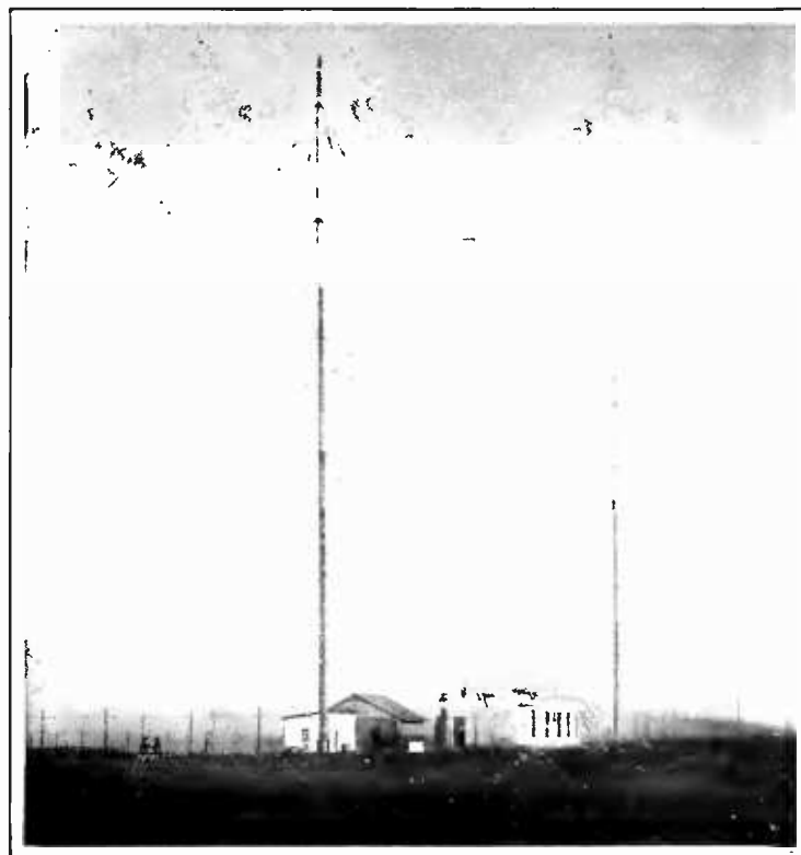
ANTENNA SYSTEM OF THE PRAGUE RADIO STATION This broadcasting station is a standard Western Electric 5 kw. outfit. The antenna is described as an Alexanderson type with three leads
