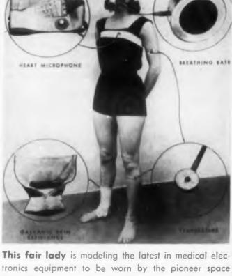
This fair lady is modeling the latest in medical electronics equipment to be worn by the pioneer space pilot. The equipment will be incorporated into space suits to outfit the well-dressed space traveler.
