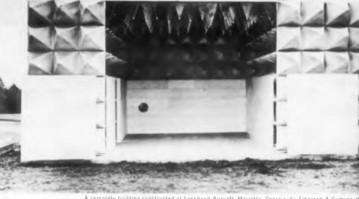
A complete building constructed at Lockheed Aircraft, Marietta, Georgia, by Emerson & Cuming II Absorber is Eccosorb CHW 570 useful from below 100 mc thru microwaves
