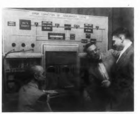
Code system to correct error bursts in digital transmission.
