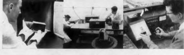
**HEAT TEST** subjects components to specified temperatures ranging from +25°C to +550°C in a heat chamber.
