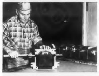
Following curing period, the mold is quickly unbolted and the Epon resin-potted transformer removed.
