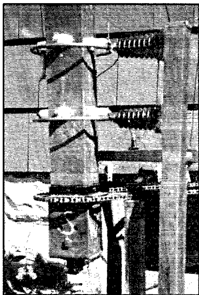
VIEW OF THE DRIVE MECHANISM AND FEEDER CONNECTORS OF THE W8ECP ROTARY ANTENNA SYSTEM
