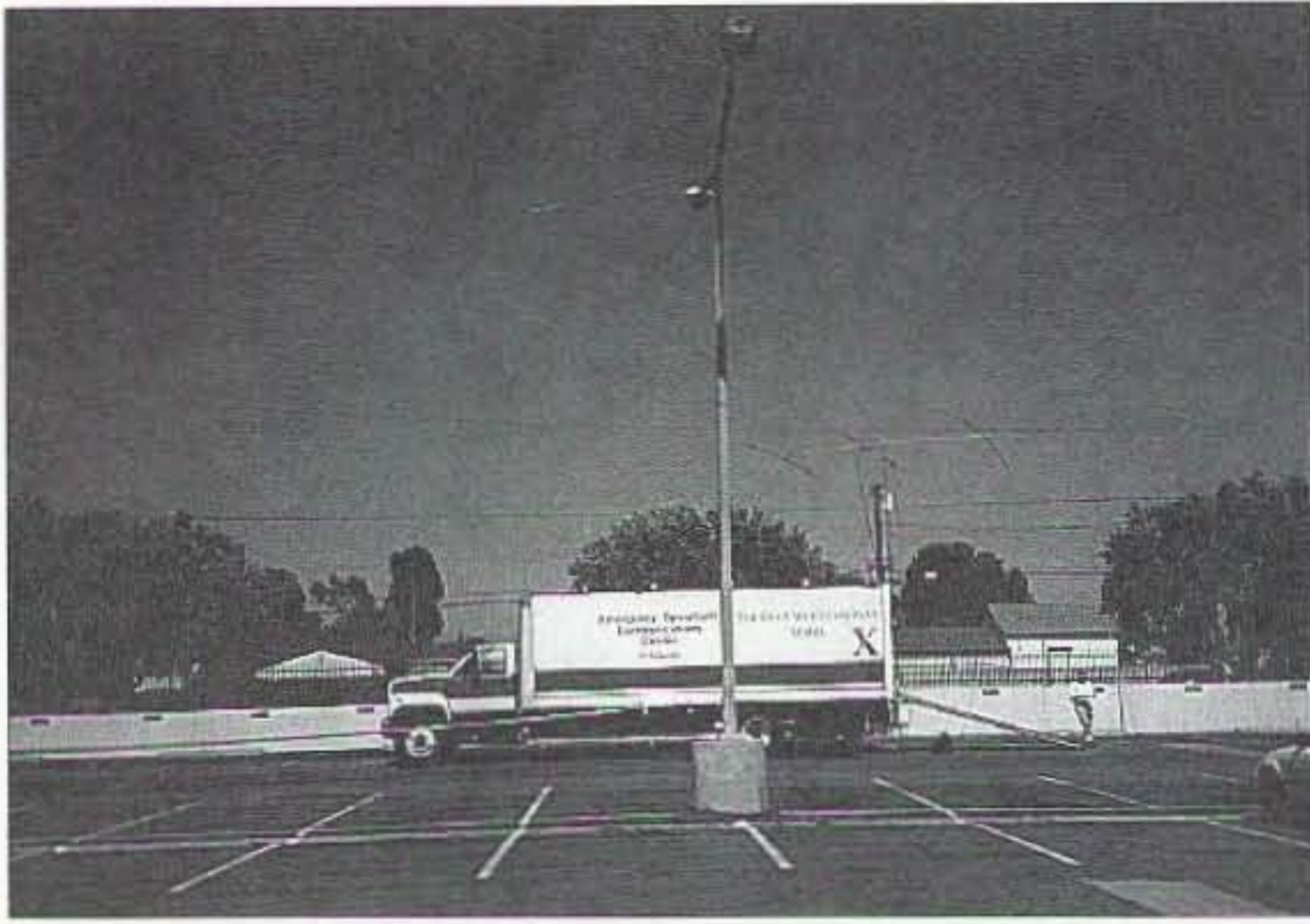
Photo G. These antennas are up and operating.
