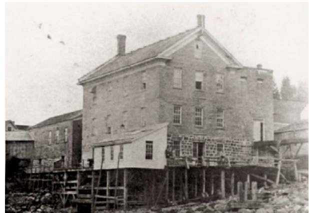
The Brick Mill, a flour mill in the converted paper mill was constructed on stilts, likely to mitigate the impacts of flooding, 1870
