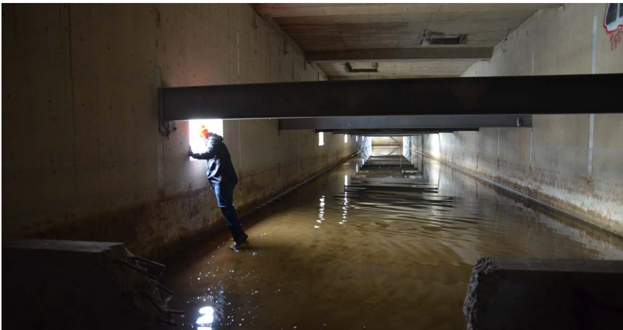
Inside the Pipe Chase
