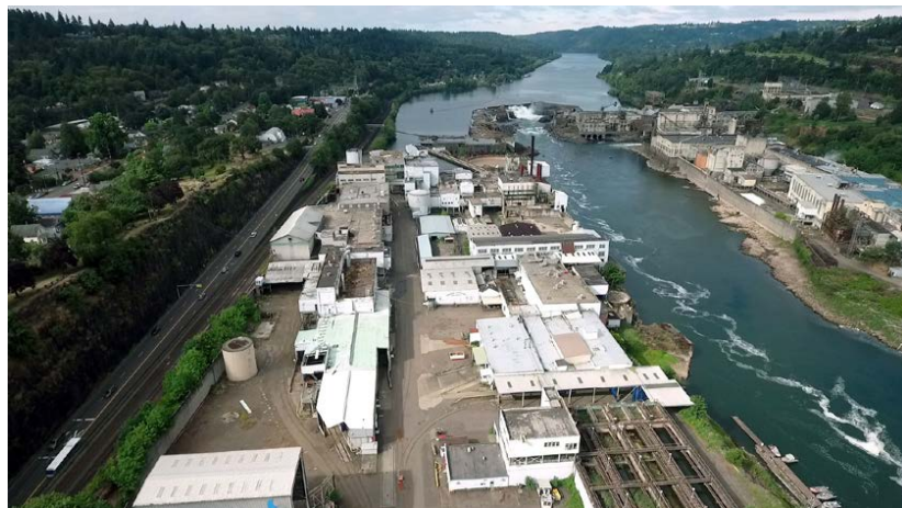
Aerial drone footage of the former Blue Heron Paper mill
