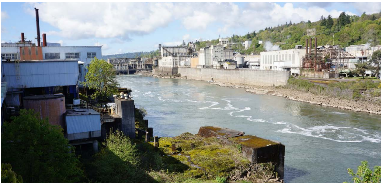
Upper Right: Oregon City Municipal elevator
