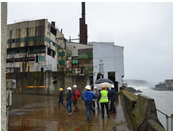
The Service Yard, standing on the Pipe Chase looking at the Boiler Plant complex
