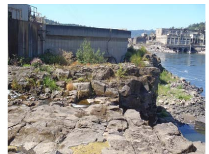
Basalt surrounding the Clarifier on site
