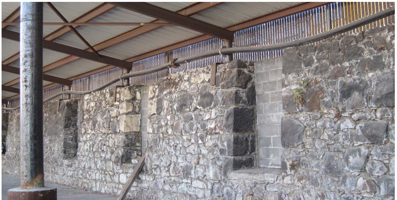
Woolen Mill basalt stone foundation walls
