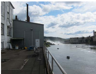
Willamette Falls viewpoint from the top of the north end of the Pipe Chase
