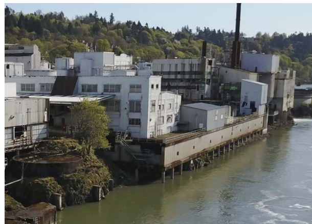
The former mill is flanked by the river on the west and the bluff along the eastern edge of the site
