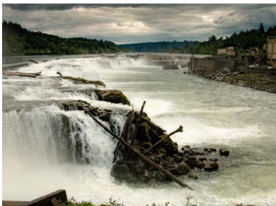
View from the Hawley Powerhouse Foundation
