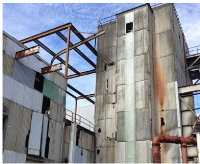
Mill H building
