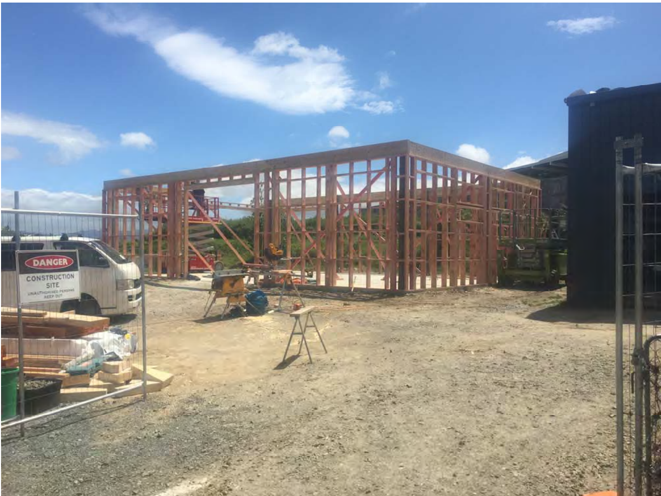
Photograph 1. – The current site and build of the proposed premises.
