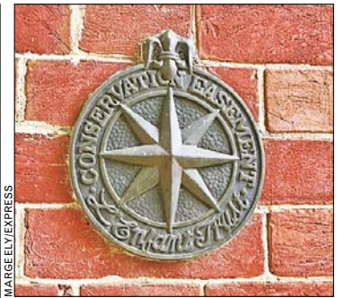
Even a building's brick walls are a concern of the condominium board's.
