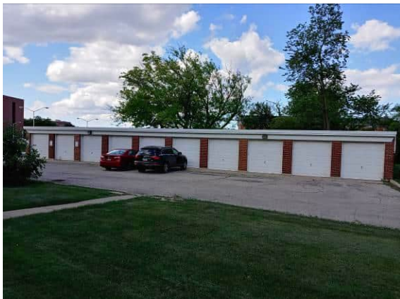
Photo #3: Typical Site garage (Building 32)
