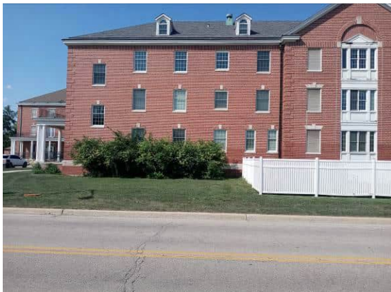
Photo #17: West adjoining VA Resources Information Center (VIREC)/Building 18 across Tripp Avenue
