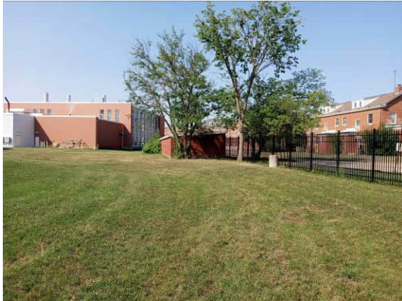
Photo #13: South adjoining boiler plant
