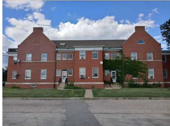
Photo #2: Former Site Apartment House (Building 24)
