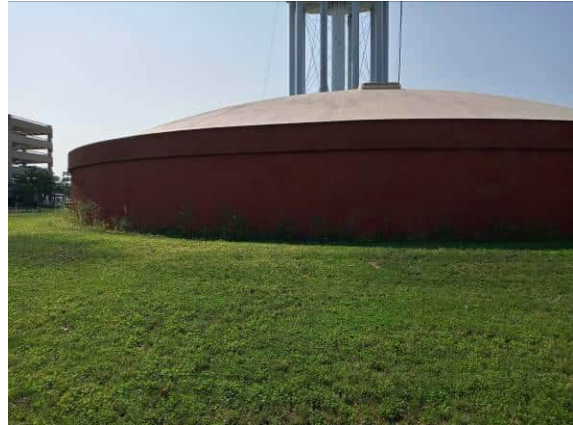
Photo #14: South adjoining water aboveground storage tank
