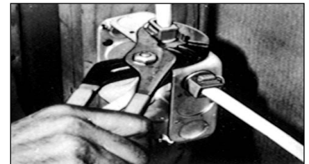
Press locking wedge into cavity which locks onto cable.
