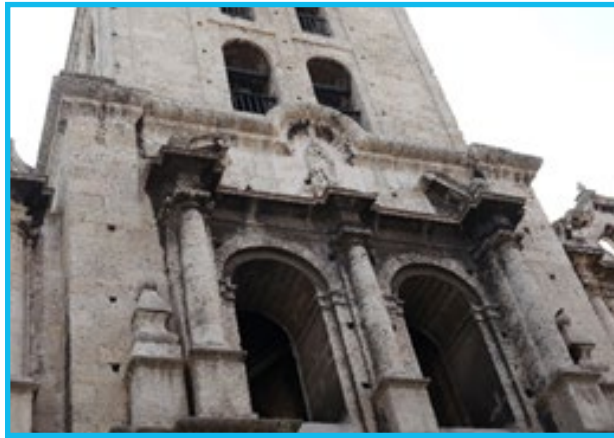
Fig. 75: Deposition of particles under cornices. Convento de San Francisco de Asís
