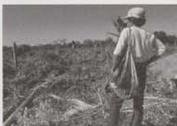
Clearing land for development.
