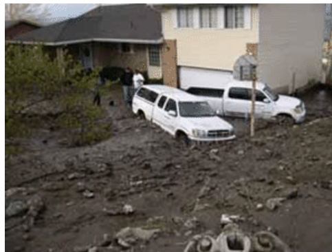
House damaged by the April 6, 2004 debris flow in Farmington, Utah.
