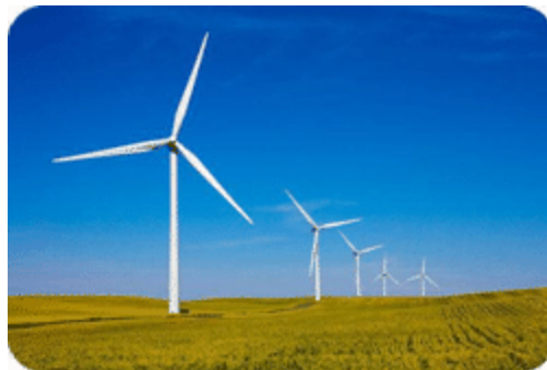
Wind power, a renewable resource, shown here in a modern wind energy farm.
