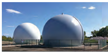
Double Membrane Biogas Holder from JDV Equipment Corporation
