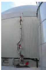
GasMix digester mixing system from Landia
