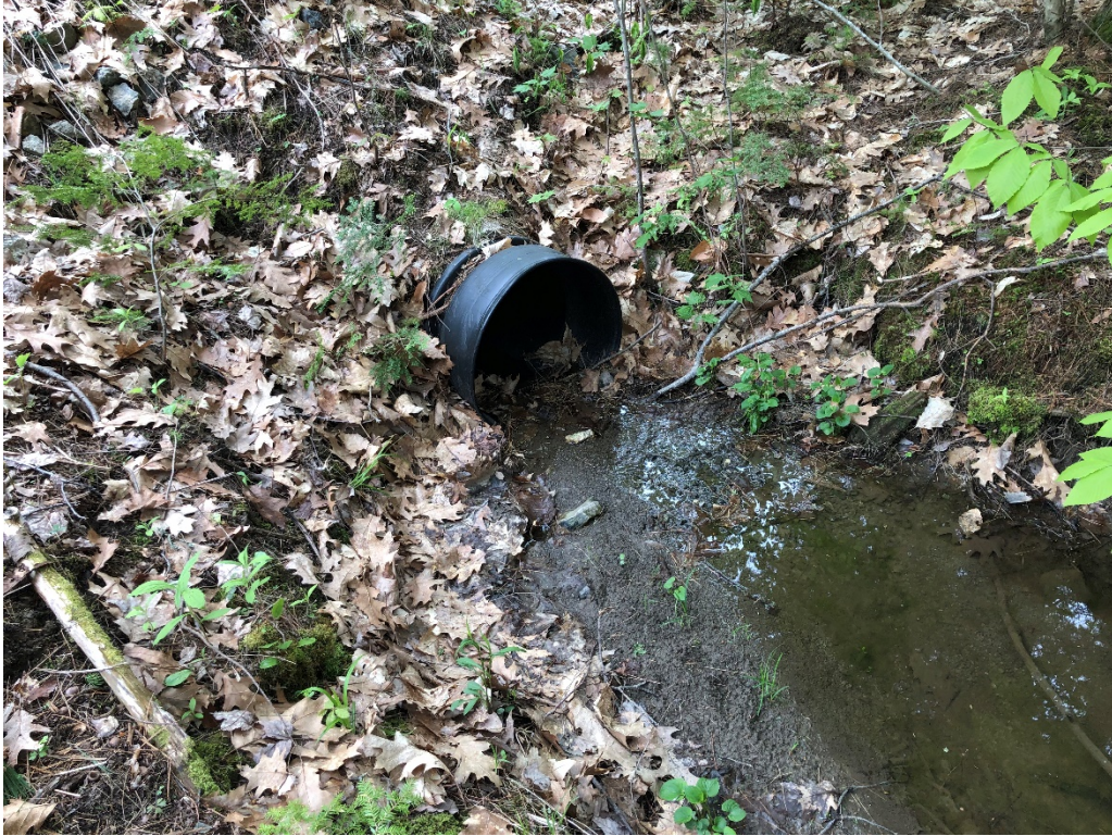
Existing Culvert at End of Redpoll Drive Sewer Extension
