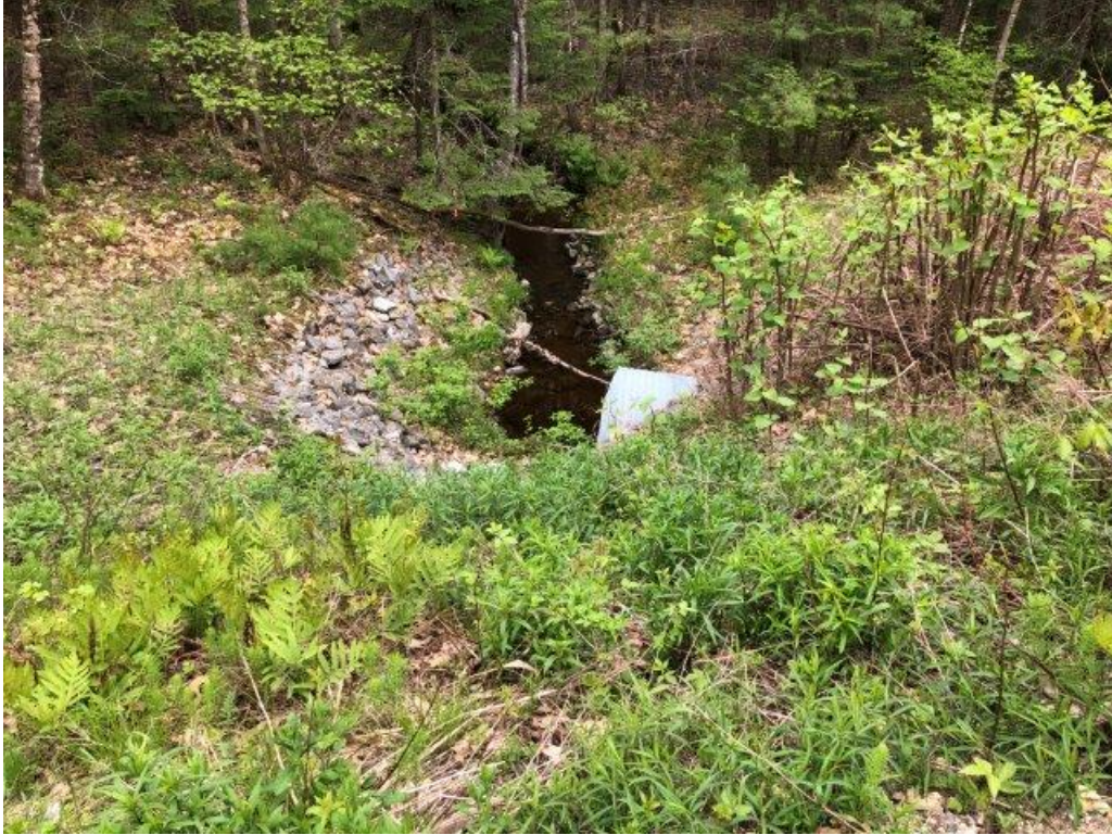
Audubon 42" Culvert Outlet
