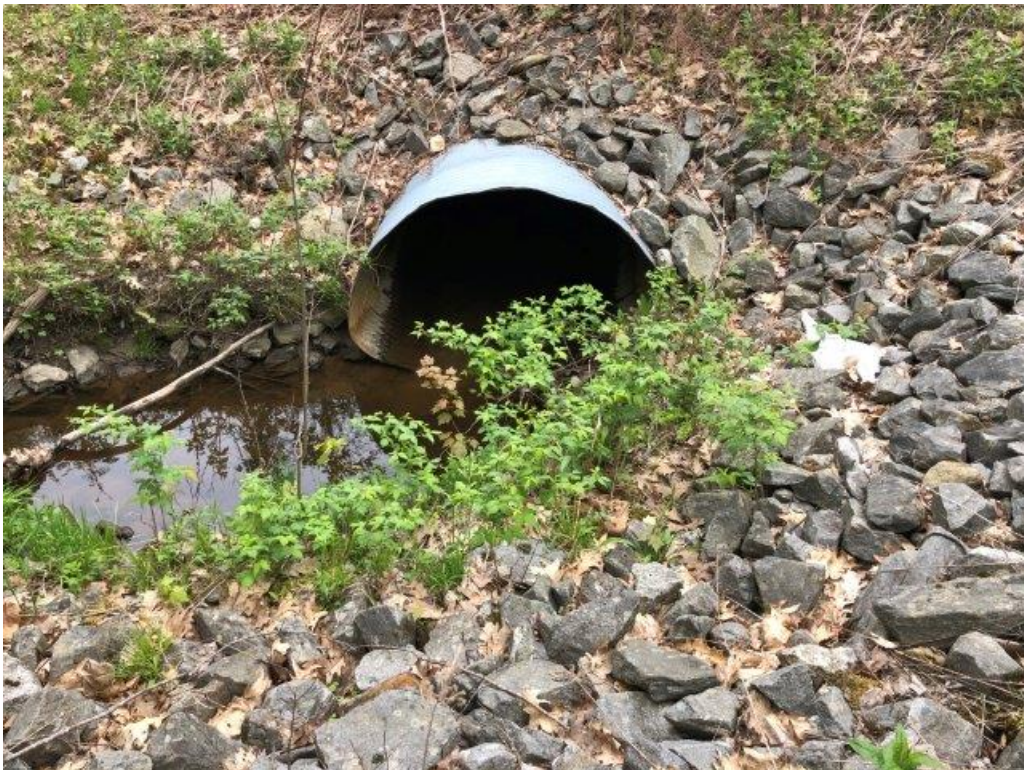
Audubon 42" Culvert Inlet
