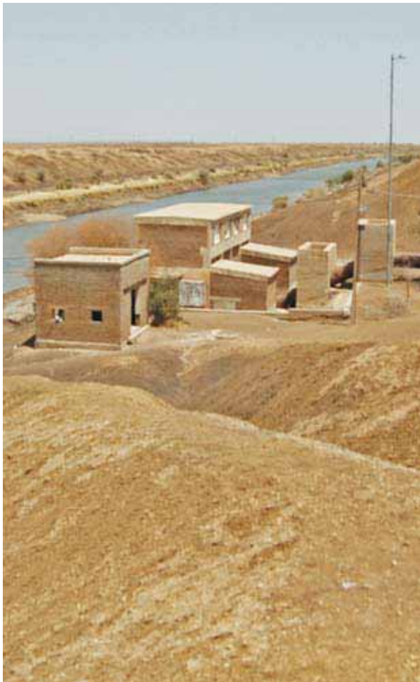
Pumping stations supply drinking water from irrigation canals that are susceptible to contamination from aerial pesticide application, such as this one in Deim el Masheihk on the Managil extension of the Gezira scheme
