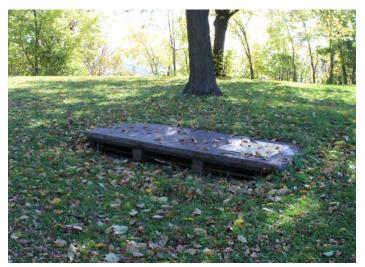
Figure 3.10. Inlet within the picnic area drains water from the perched wetland soils (QEA, 2018).
