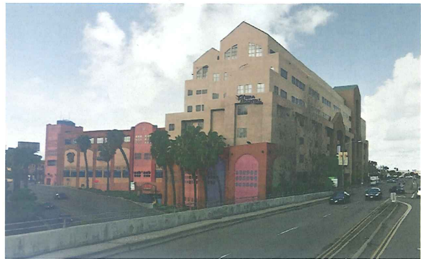
East Elevation from Washington Street
