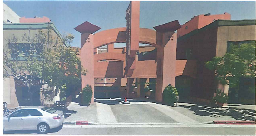
West Elevation at Parking Garage Entrance
