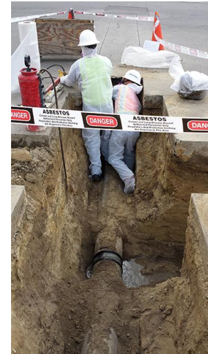
Proper asbestos pipe removal and disposal by a Casper Company for TC on MACC 1, Task Order 1, Skyline Avenue in front of Morse High School.
