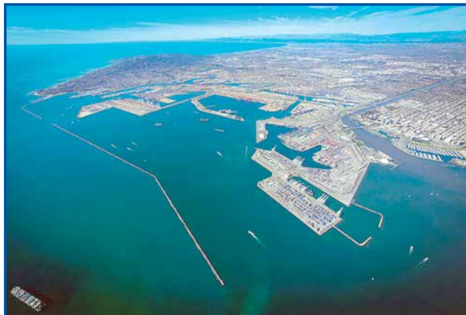
San Pedro Bay Ports Aerial
