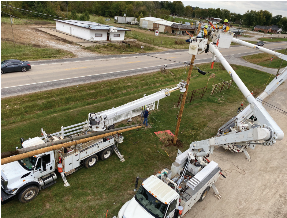
A crew of Kelly Eck, Randon Marshall, Rodney Williams, and Brian Fugate perform a pole replacement overlooking 54 highway.
