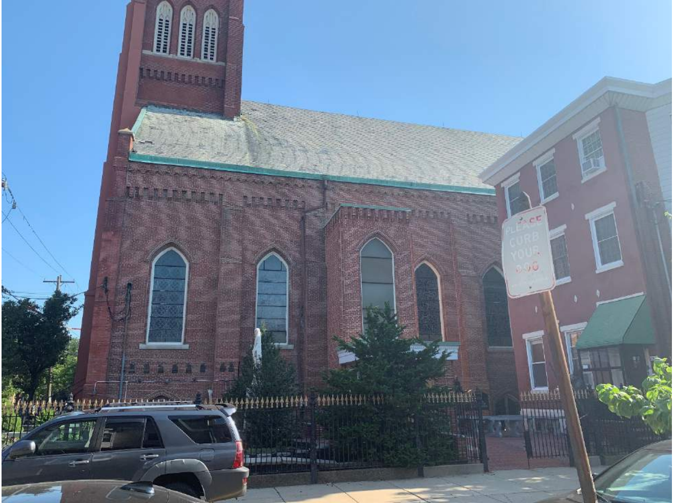
South (side) elevation, view from Greenwich Street, July 2019.
