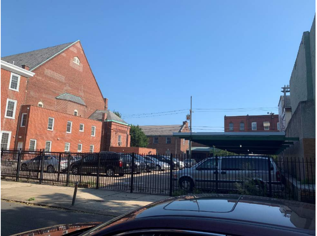
East (rear) elevation of church with gable roof, also showing non-contributing carport at edge of parking lot. View from Greenwich Street, July 2019.
