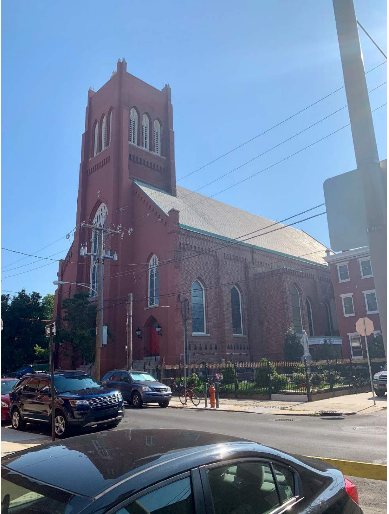
Primary and south façades from S. 10 th and Greenwich Streets, July 2019.
