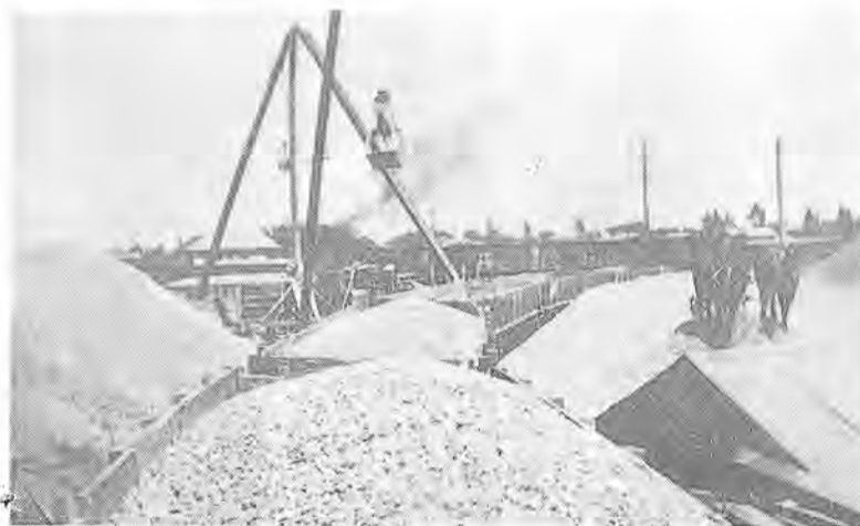
TRAIN LOADING —with no identification on this shot, it looks like a clam bucket and stiff-leg arrangement to load rock into nearby trains in the Lindsay, Calif. area in 1923. Note team of horses at right keeping stockpile level.
