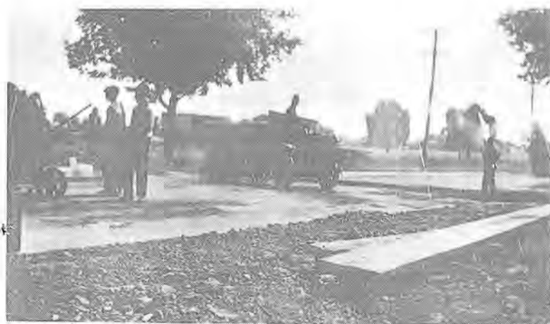
EARLY TRUCK —Brother Les Nedrow, now living in Stockton, wheeled this early two-cylinder Autocar truck in Lindsay, Calif. Workers at left are shown heating rakes to lay "hot stuff" by hand. The truck carried one ton of material. Contrast with today's modern, automatic behemoths capable of a 100 tons and more, and the modern slip-form paver to lay asphalt.
