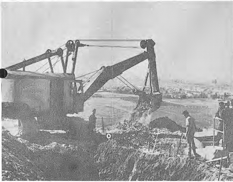
HILLTOPPER —this P & H three-yard backhoe is shown above and below on a hillside in Livermore Valley area. Operator is George Curts and lube engineer Joe Carney. Note the "sled" constructed to keep the shovel level during operation. It is pulled backwards down the hill by a dozer, while digging trench for San Antonio-Calaveras pipeline nearly two miles in length.
