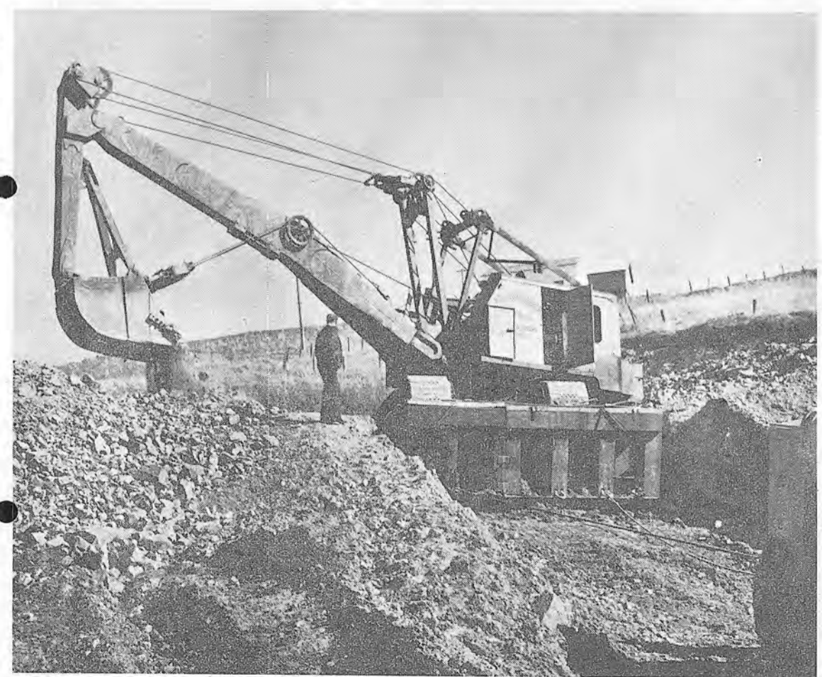
HILLTOPPER —this P & H three-yard backhoe is shown above and below on a hillside in Livermore Valley area. Operator is George Curts and lube engineer Joe Carney. Note the "sled" constructed to keep the shovel level during operation. It is pulled backwards down the hill by a dozer, while digging trench for San Antonio-Calaveras pipeline nearly two miles in length.
